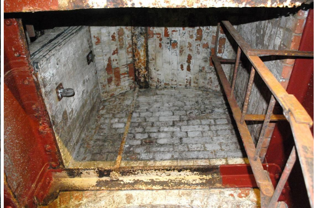
Fig. 29 (above): View upwards into ceiling space at B/C-14 from west, showing end of trimmer joist to opening , also pulleys for former control cables.
