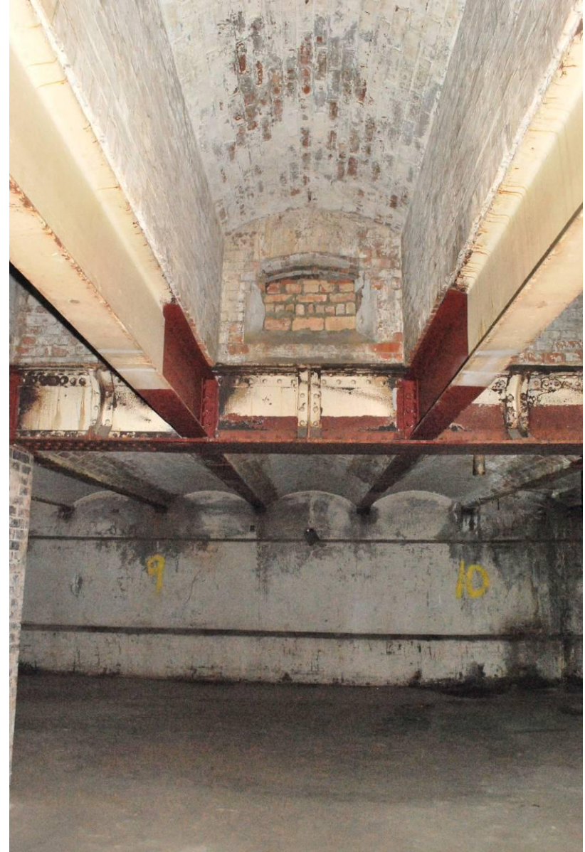
Fig 18 (above): View southwards at E side of Basement, with back of former retaining wall on left. Main beam (north-south) with brick-encased columns. Secondary beams (east-west) beneath former rail track.
