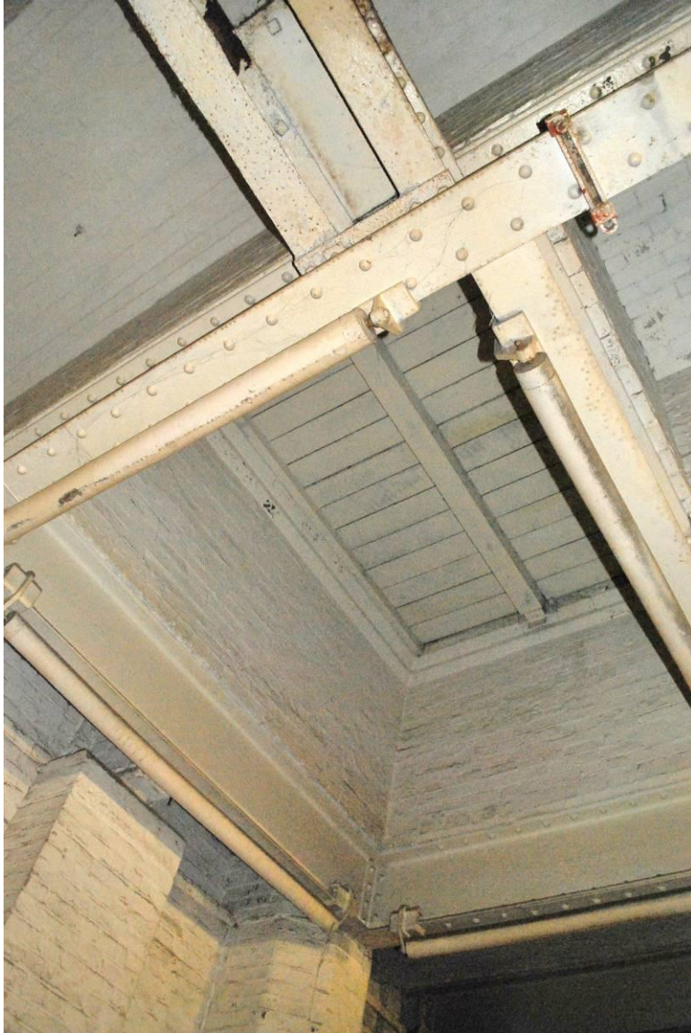
Fig 25 (above): Detail of rollers below trap door to protect against wear from ropes.
