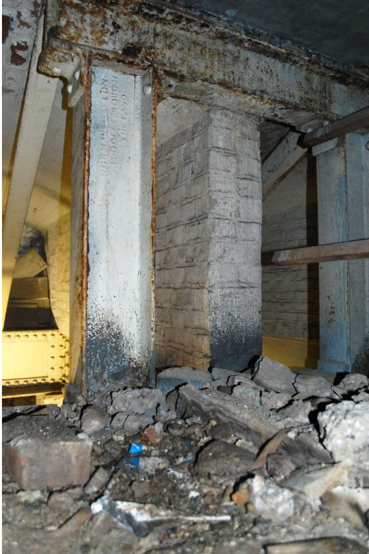
Fig. 29 (above): View upwards into ceiling space at B/C-14 from west, showing end of trimmer joist to opening , also pulleys for former control cables.
