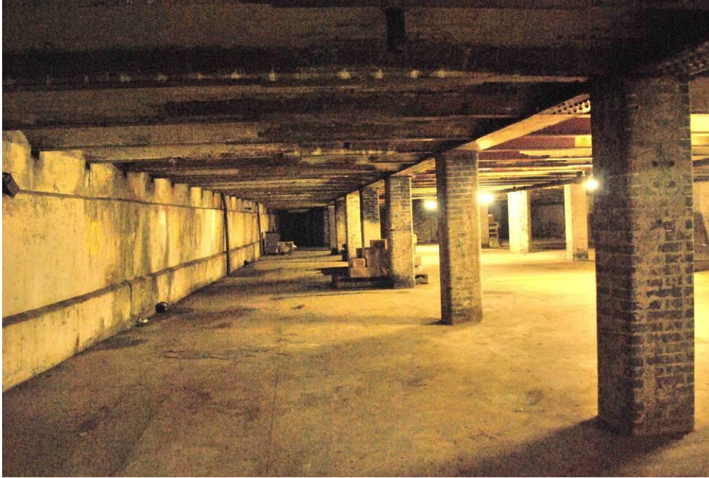
Fig 18 (above): View southwards at E side of Basement, with back of former retaining wall on left. Main beam (north-south) with brick-encased columns. Secondary beams (east-west) beneath former rail track.
