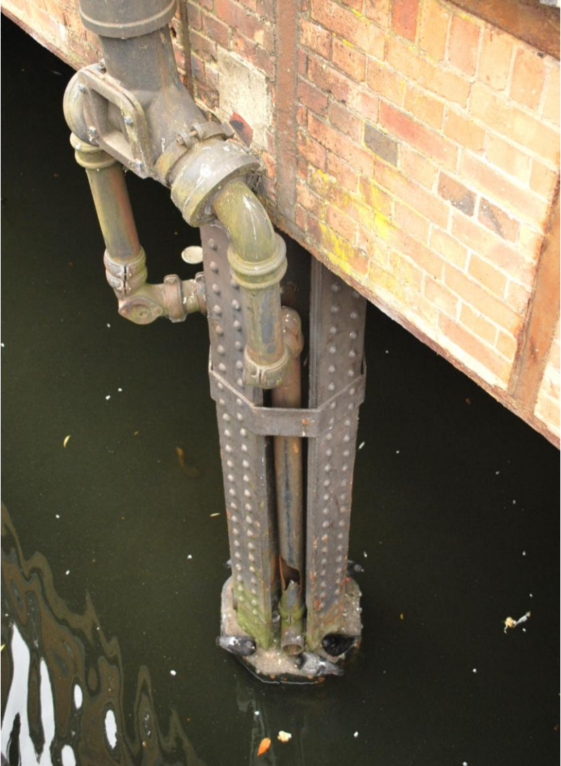
Fig. 17: Cruciform Steel Column at Dock Entrance.
