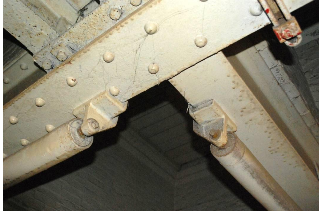
Fig 25 (above): Detail of rollers below trap door to protect against wear from ropes.
