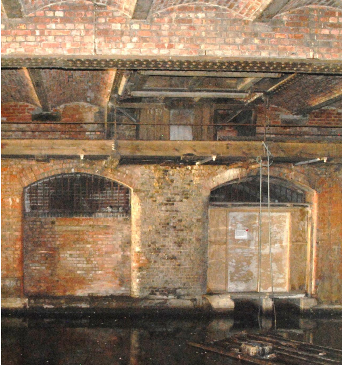
Fig. 38: Ceiling over Dock at E/F-6, showing trap door and suspended mounting for a platform crane, with north-south crawl-way for access.
