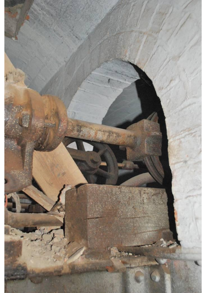
Fig. 32 (right): Slewing rams extending through the archway, viewed from SE.
