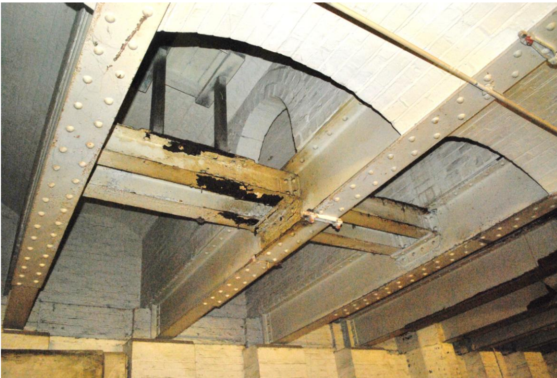
Fig. 25 (above): Twin beams to support platform crane, seen here at C/D-10. Note small square hole for foot of crane post and archway for slewing rams. View from SE. Compare Figs. 31-2.
