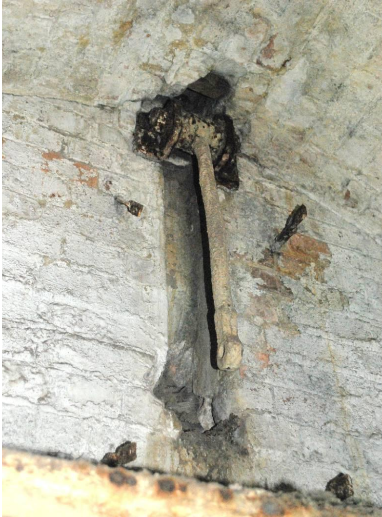
Fig. 35: Hanger bar for support of a control rod that passed through hole in platform wall behind. (See paragraph 4.4).
