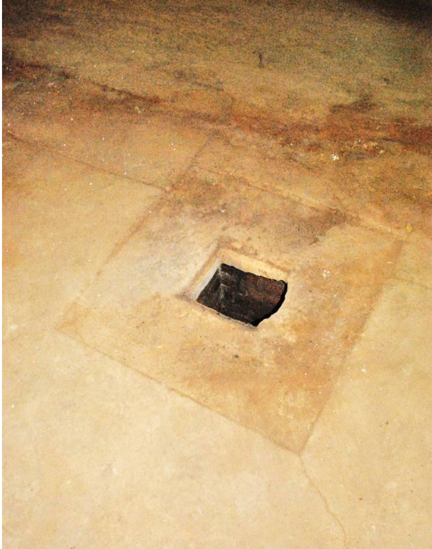
Fig. 22 (left): Drainage gully in floor
