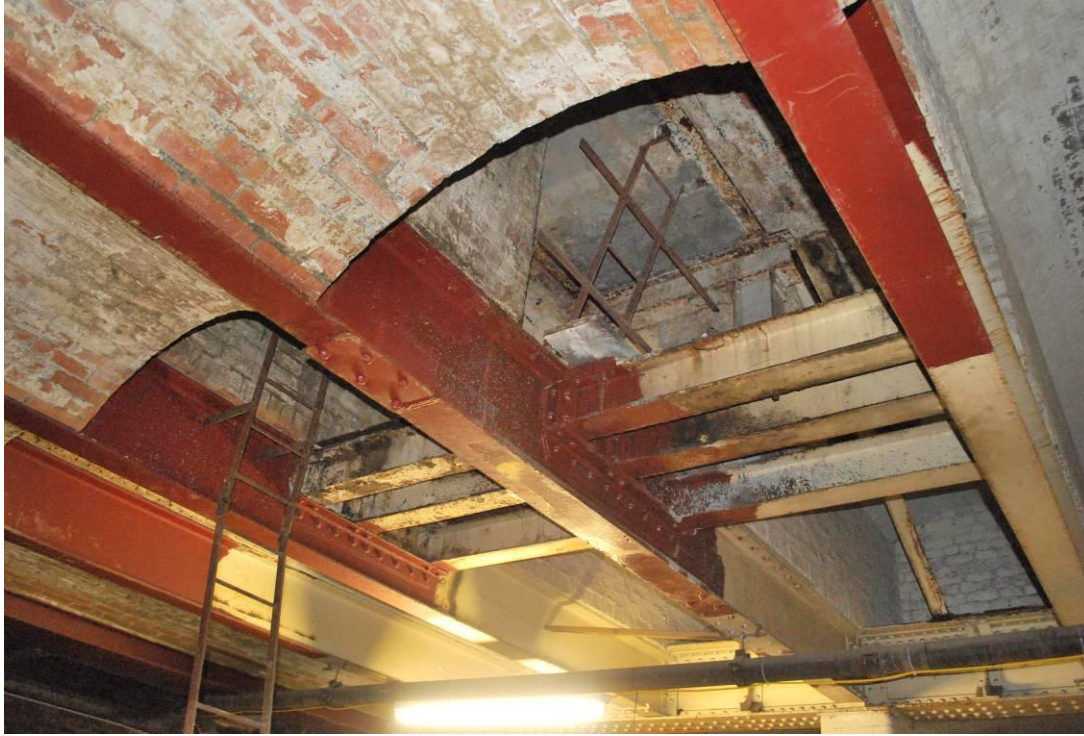
Fig. 27 (above): More elaborate mounting for platform crane at B/C-14 with third beam, viewed from NE.
