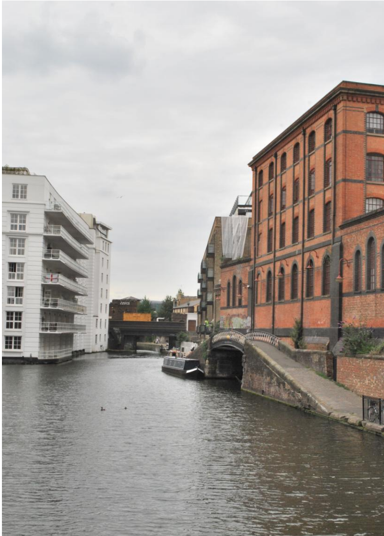
Fig. 16: Canal Frontage and Bridge over Dock from E.
