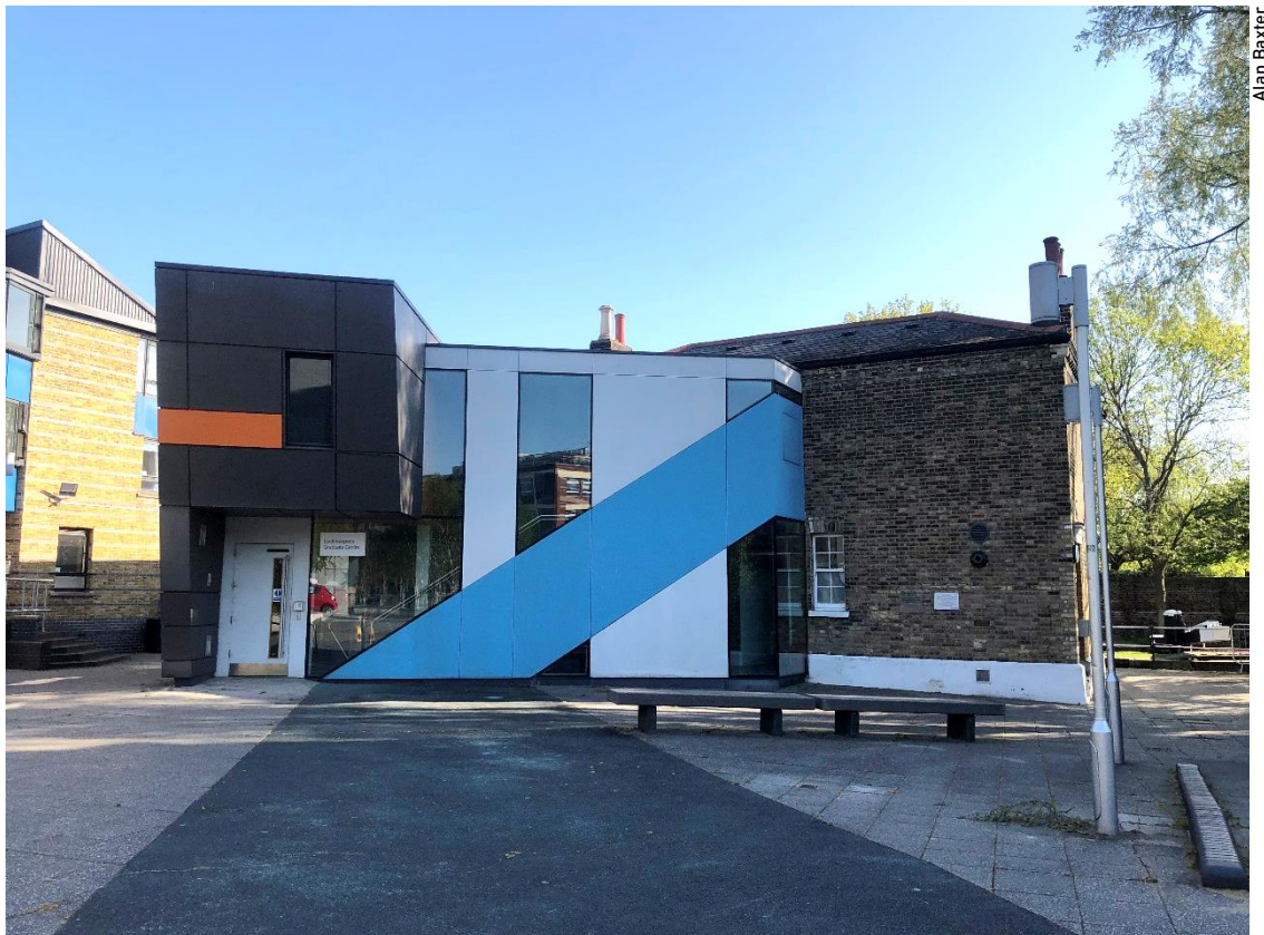
Figure 20 The west elevation of the lock-keeper's graduate centre (2020)
