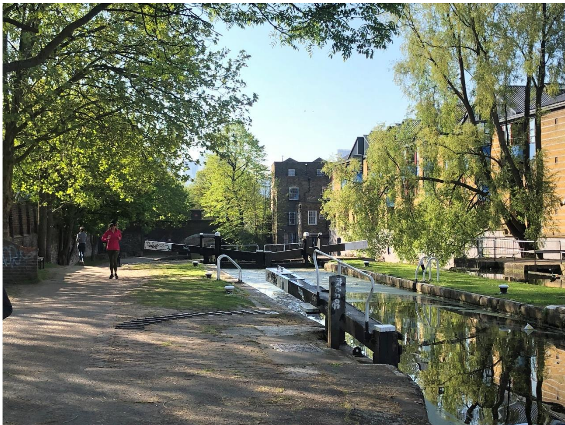
Figure 12 The rear of no. 357 and Mile End Lock looking south from the east side of Regent's Canal (2020)
