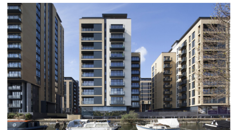
Suttons Wharf North
