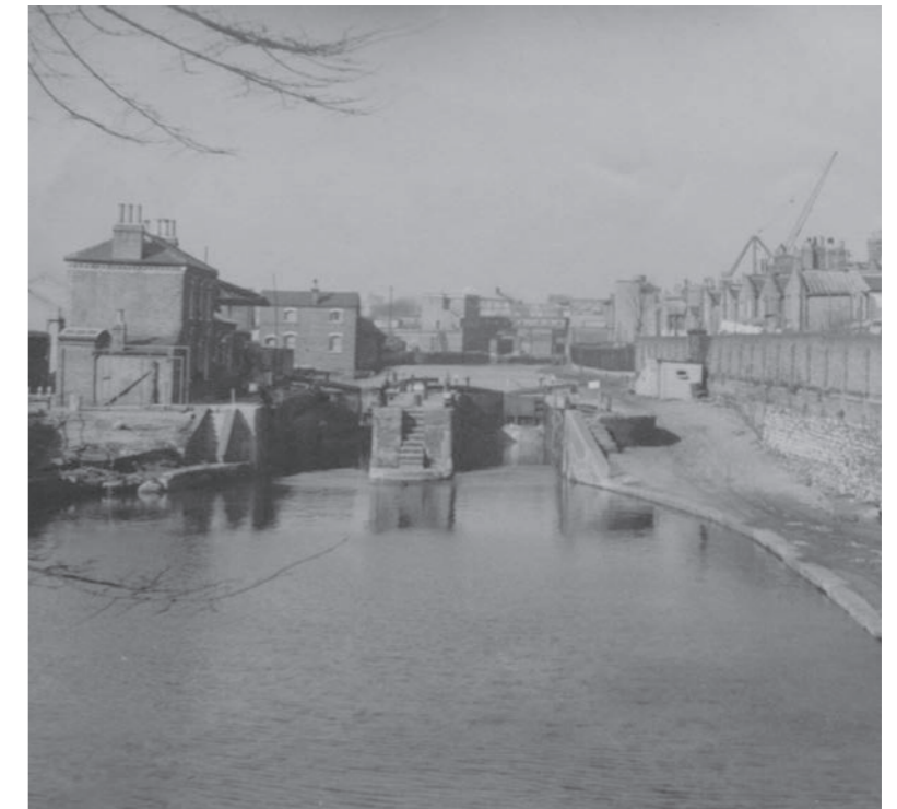
Mile End Lock basin looking north (pre-war, date unknown)
