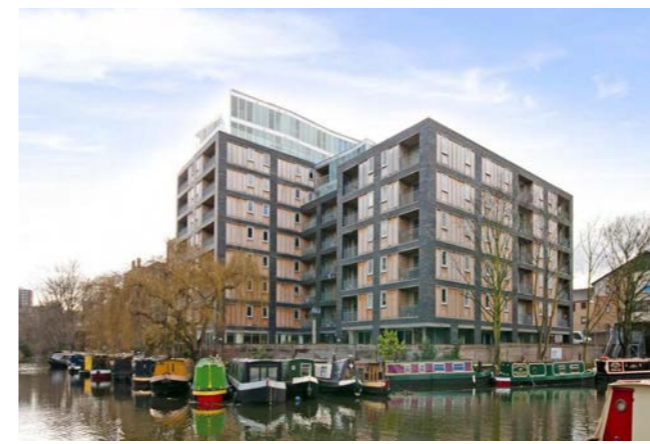
07. Wenlock Building, Islington
