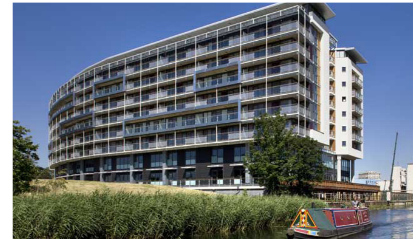
Suttons Wharf South
