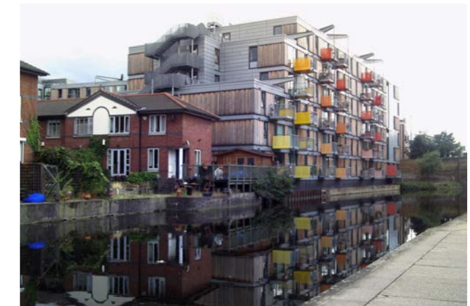
04. Adelaide Wharf, Hackney
