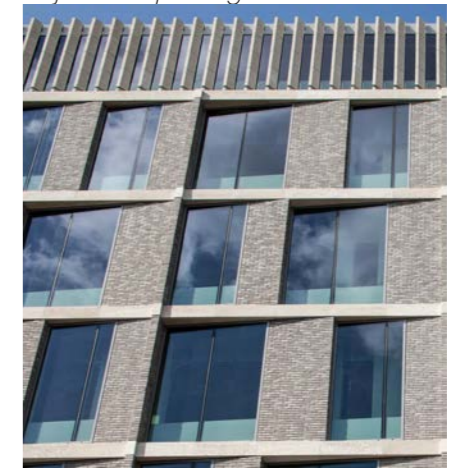
Horizontal precast banding
