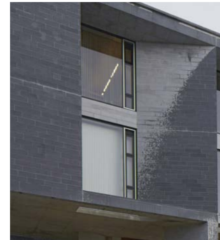
Chamfered brick window reveals
