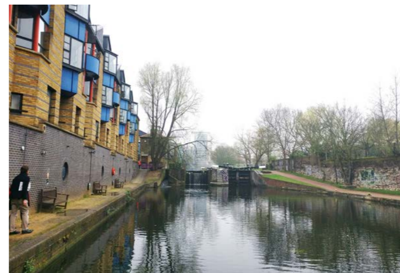
Hatton House and the canal-side path - existing condition
