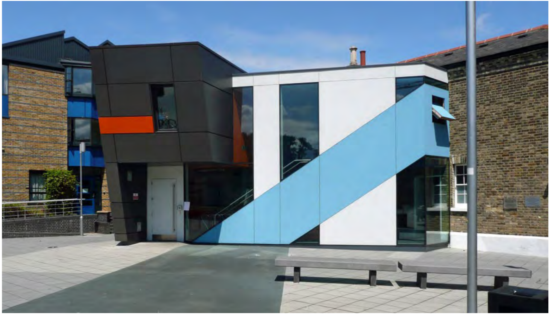
View of Lock Keeper's Cottage showing completed new extension and entrance (2006)
