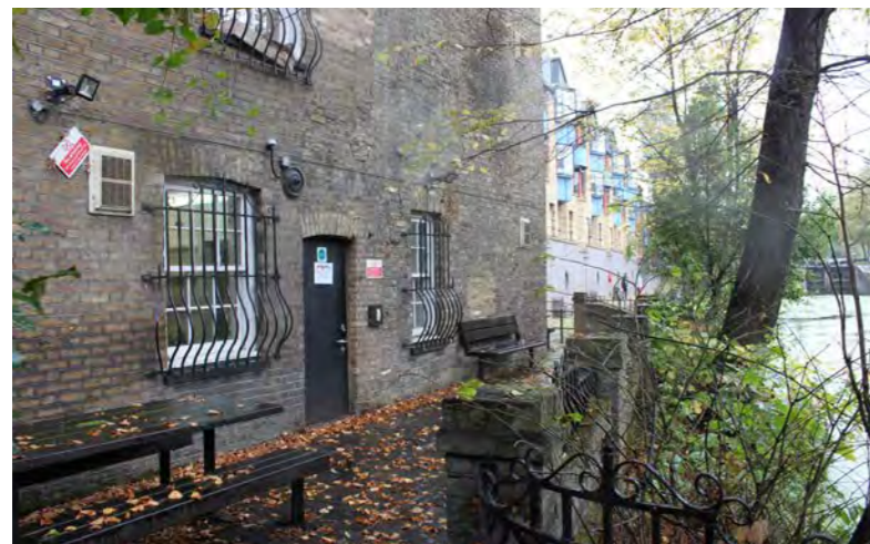
4. No. 357 Mile End Road canal elevation
