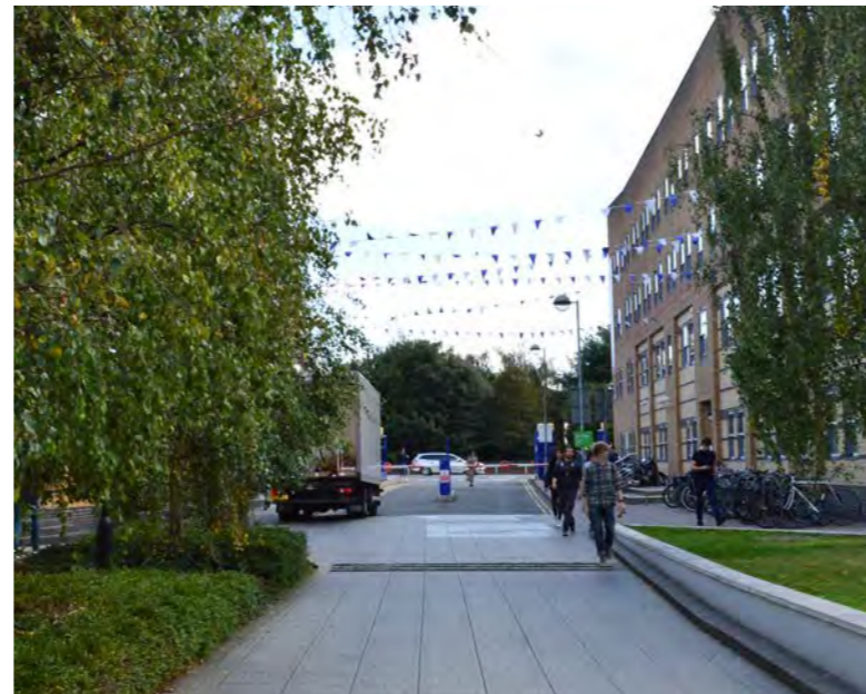
1. View of Arts 1 building, looking south
