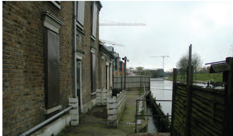
Cottage entrance (2004, prior to demolition of pump house)
