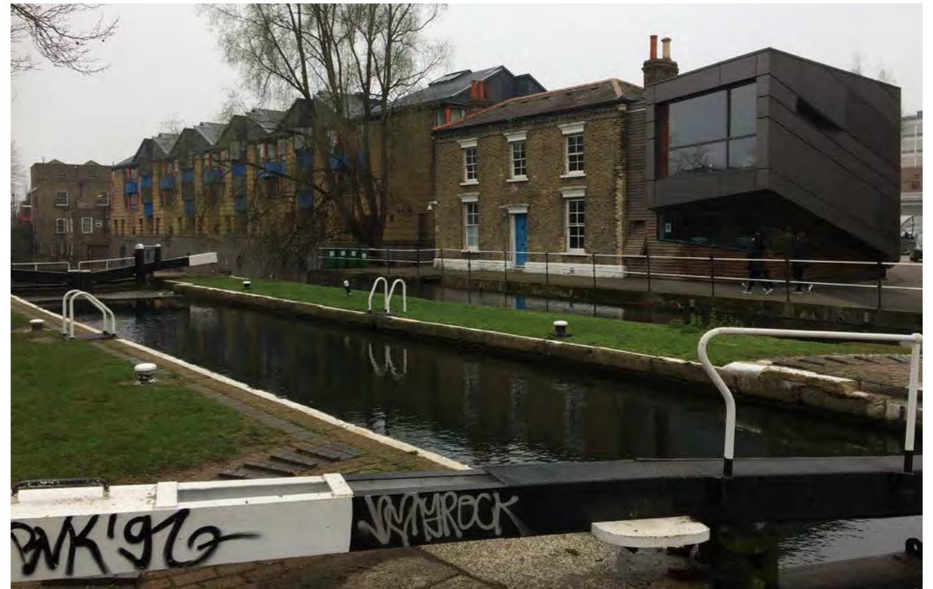
4. View of Hatton House and the lock keeper's cottage from Mile End Park
