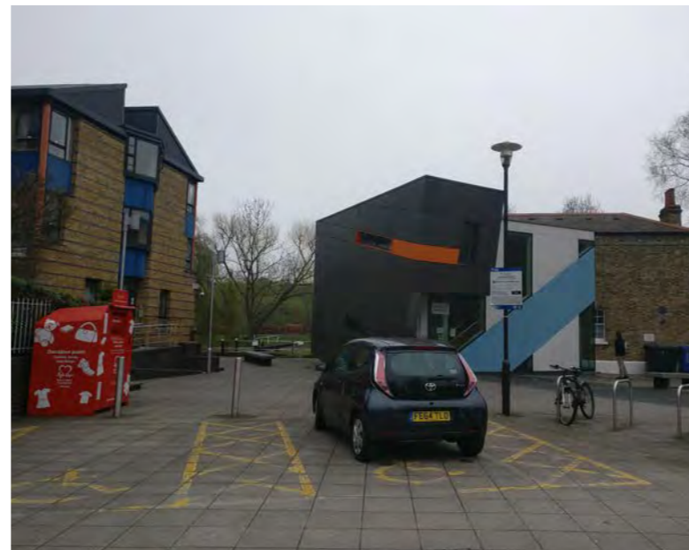
4. View of Lock Keeper's Cottage, looking north east
