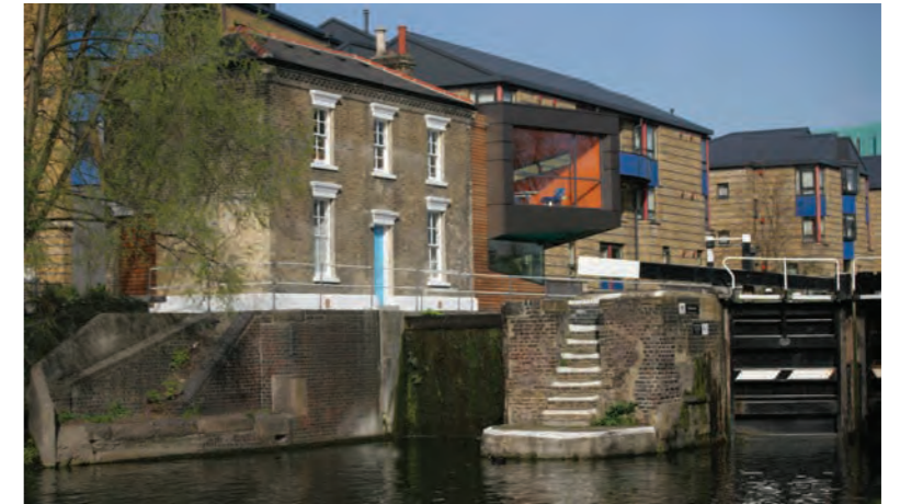
View of the lock keeper's cottage and extension (2006)
