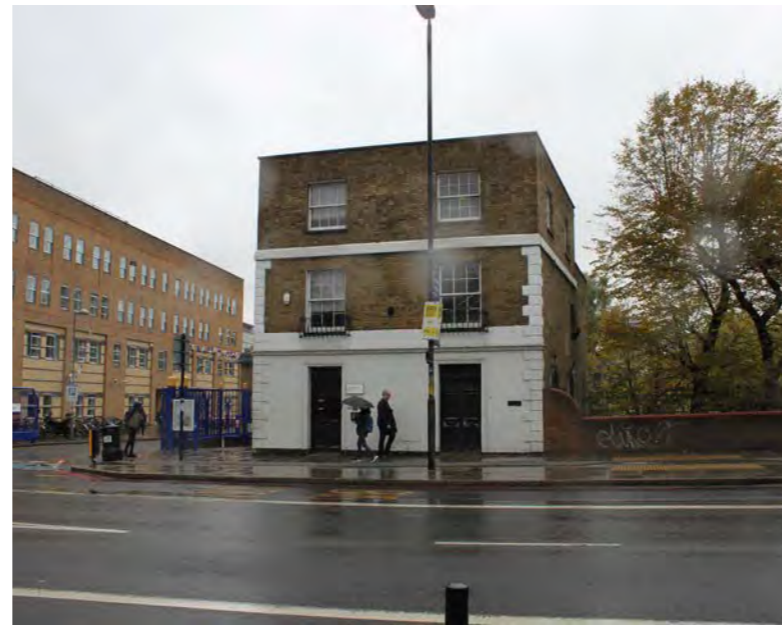
1. View of 357 Mile End Road looking north
