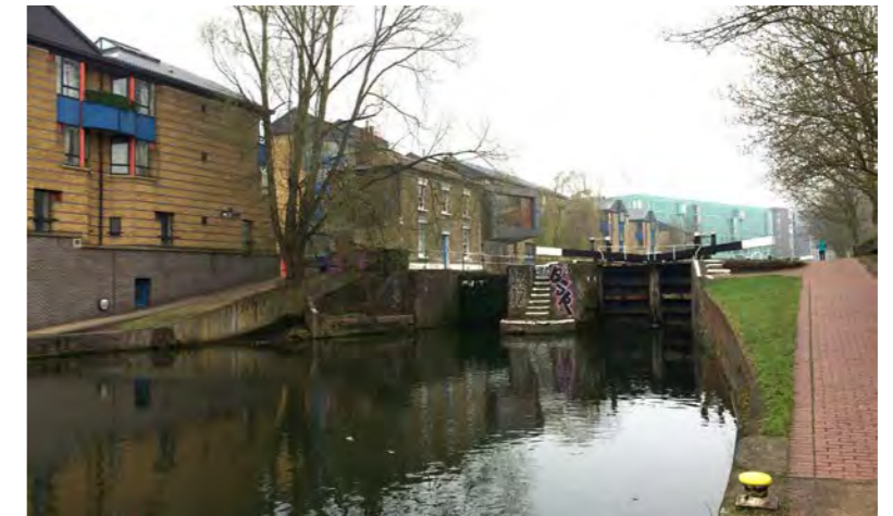
Regents canal context - Mile End Lock basin
