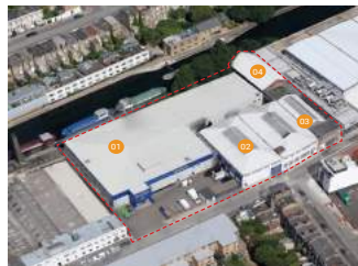
01 Light Metal Frame Building (2002) 02 Concrete Building (1937) 03 Brick Building (1940) 04 Victorian Brick Warehouse (c.1860) with Potomac Truss
