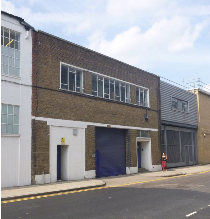
Fig. 17: Facade of 1965 building
