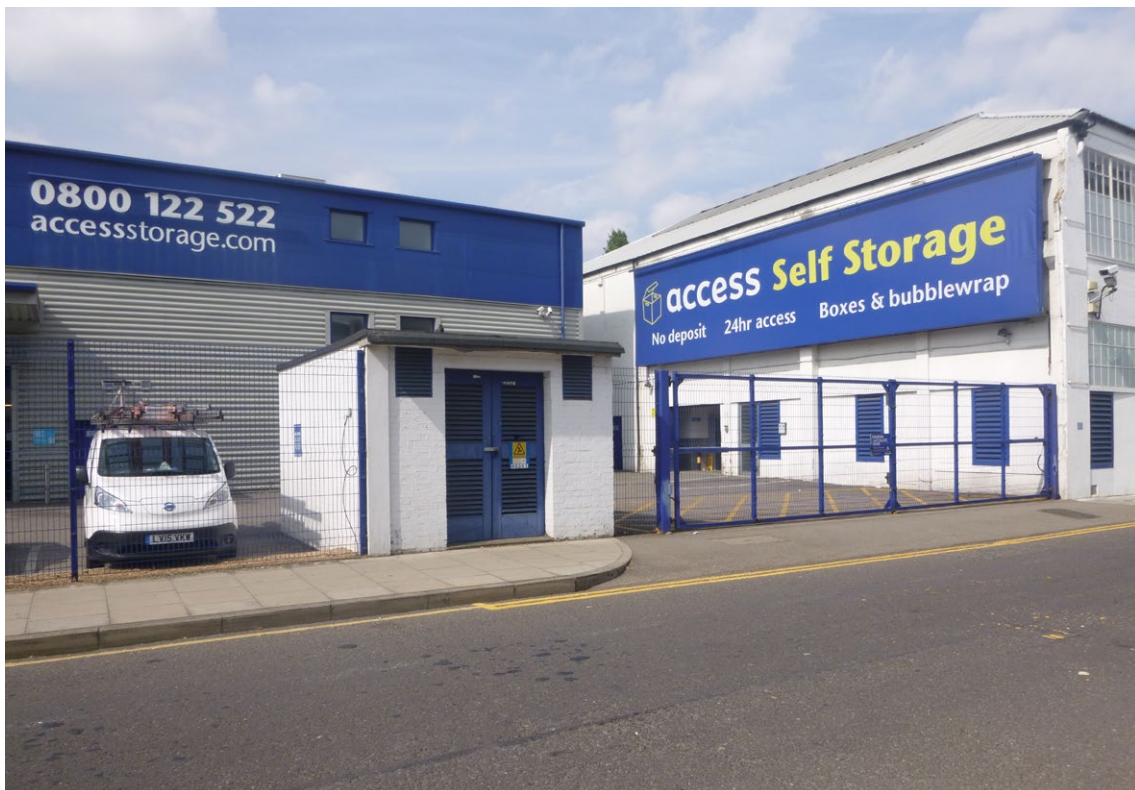
Fig. 9: Current storage building on site
