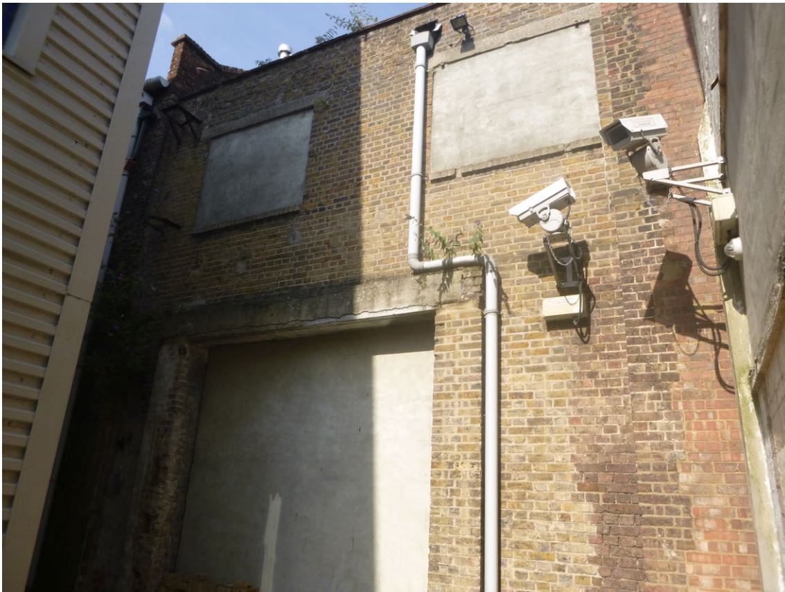
Fig. 13: Link between Victorian building and 1937 building
