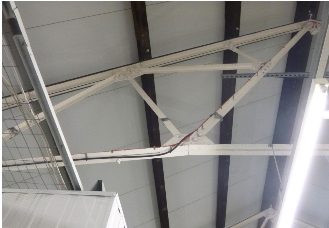
Fig. 10: Victorian building wrought iron roof trusses with modern roofing above
