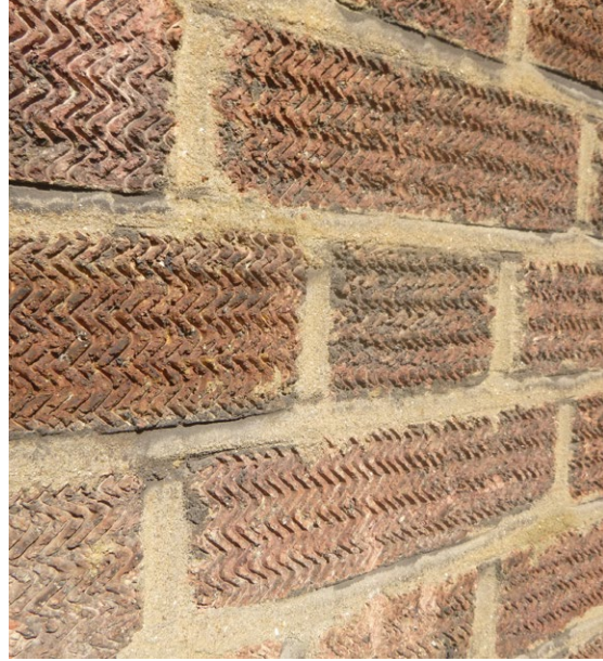
Fig. 12: Textured twentieth-century brickwork to facade of Victorian building
