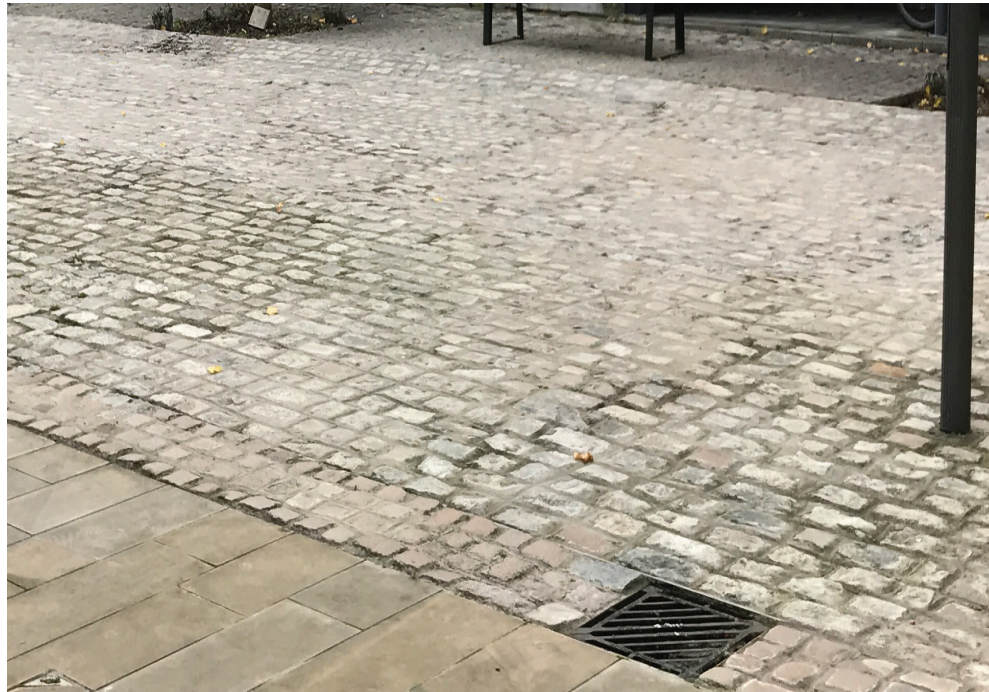
Traditional granite setts at Kings Yard, Kingsland Road
