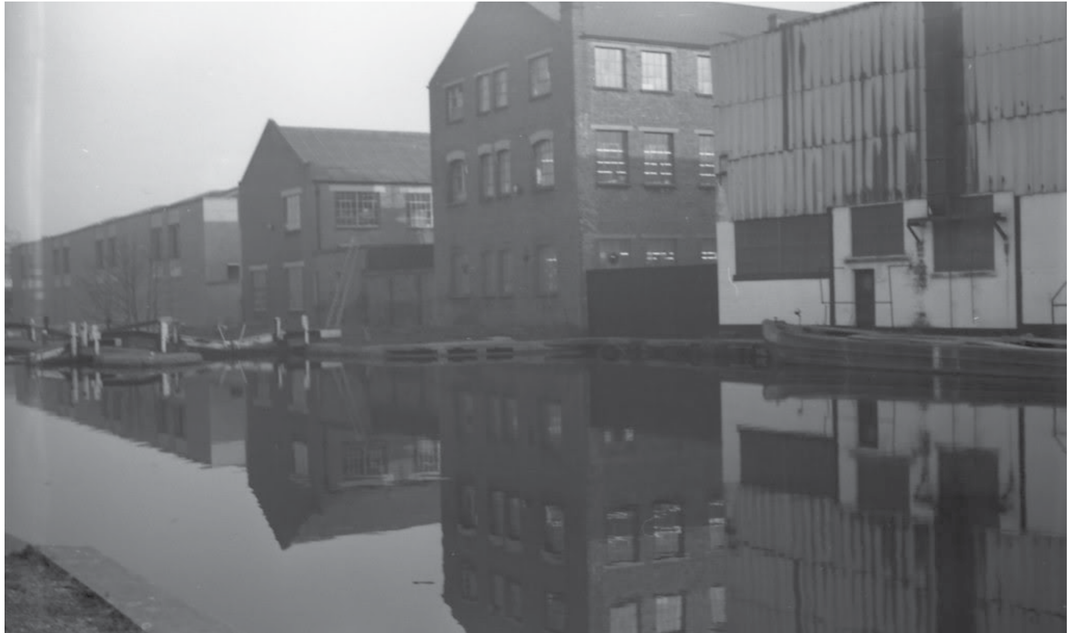
The 1871 industrial grain of 48 Eagle Wharf Road. - a pair of gabled-roofed north-south blocks with an open yard between.
