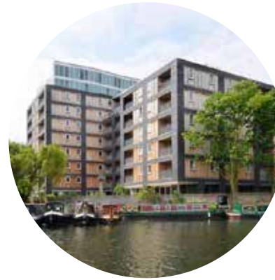
Regents Canal Wenlock Waterside Offices at Wenlock Basin Hackney Borough
