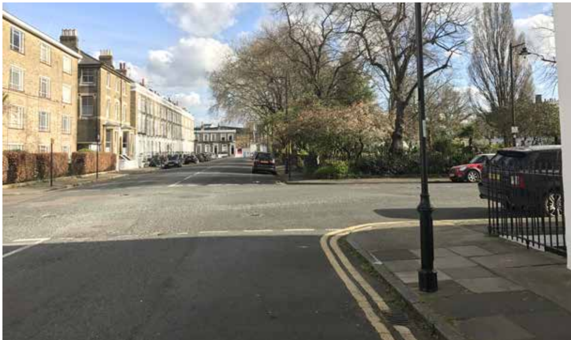
Linton Street (East) view towards Royal Mail at existing heights (centre) and Holborn Studios (right).
