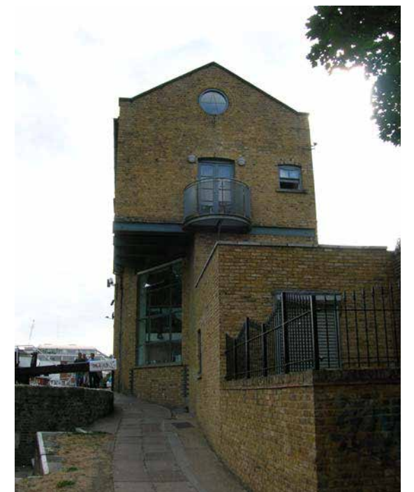
Refurbished Lock Keepers Cottage and
