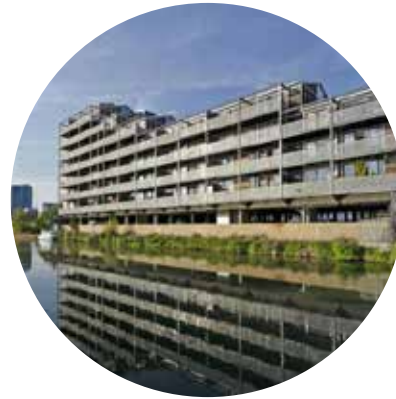
Lea River Meets City Mill River Three Mill Lane Bridge Tower Hamlets B Lt, Newham B Rt
