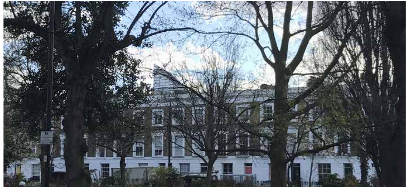
10 ARLINGTON SQUARE ROAD (EAST) VIEW TO 261 LEXICON CITY ROAD (CENTRE)
