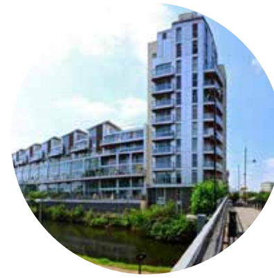
Regents Canal Roman Road Bridge Tower Hamlets Borough
