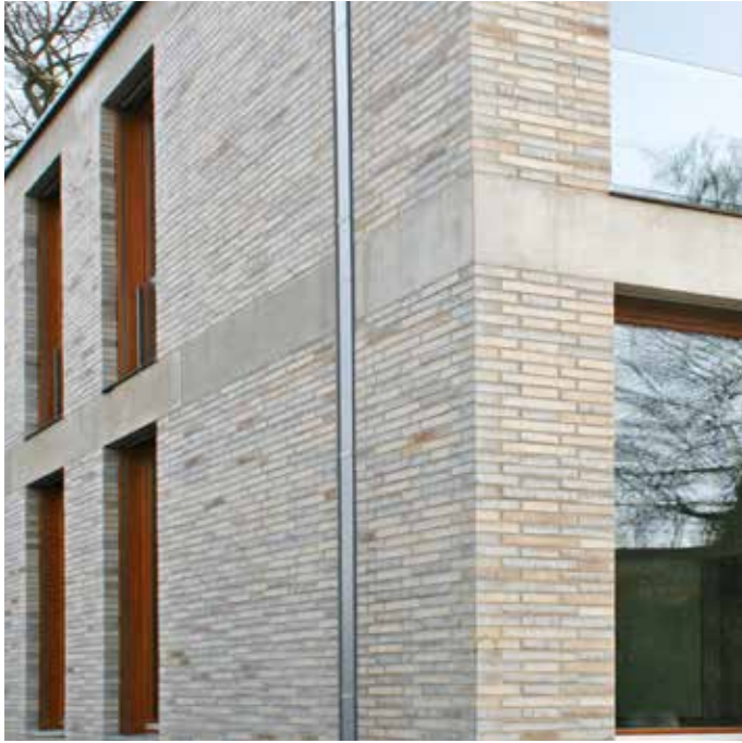
M51 Shadow gap with rainwater downpipe
