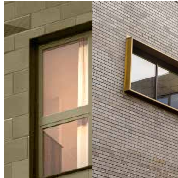
M16 Projecting copper window surrounds
