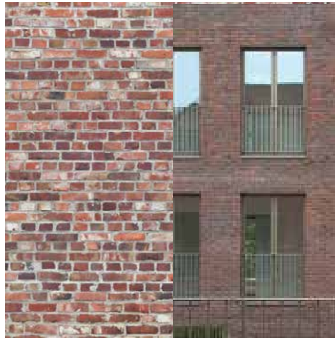
M02 Variegated red, pink, rose multi-stock brick blend, variegated coursework and brick relief detailing
