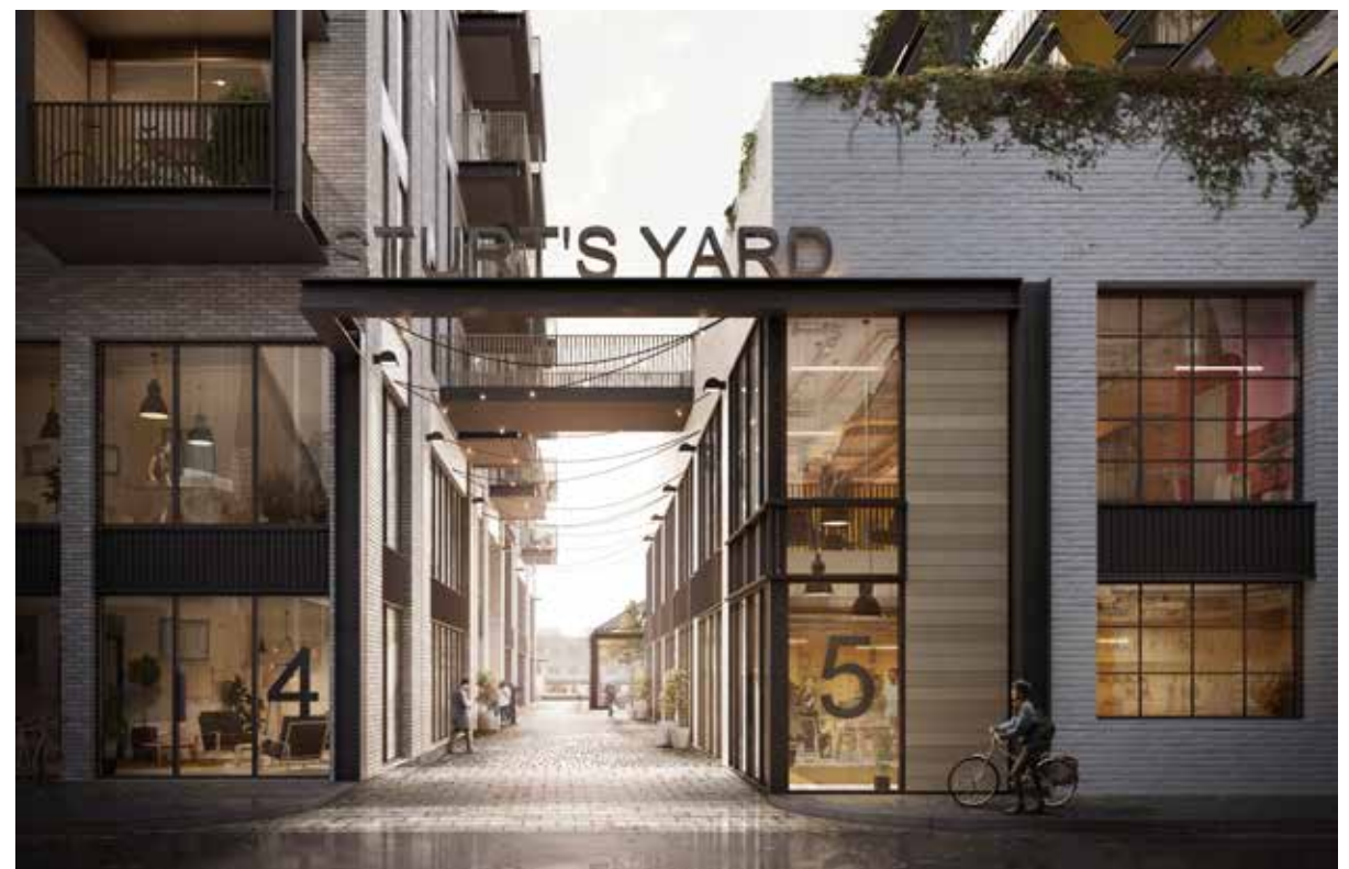
Northern passage from Eagle Wharf Rod to Regent's Canal and Sturt's Yard
