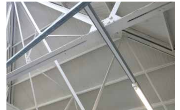
1937 Build Roof Trusses
