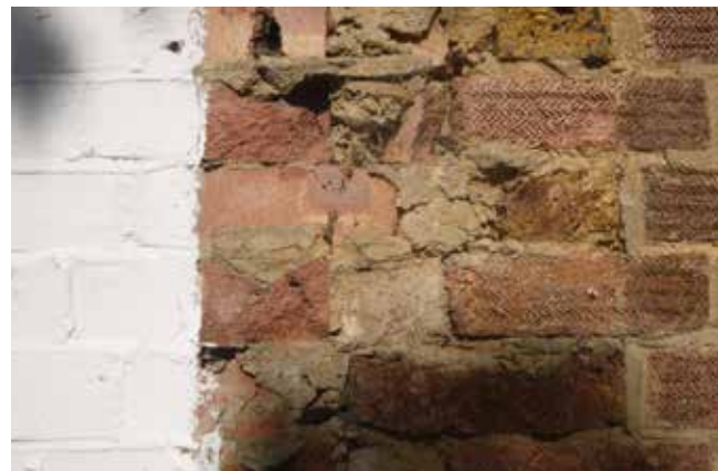
Patchwork repairs to Victorian building
