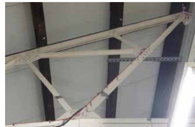
Victorian building wrought iron roof trusses
