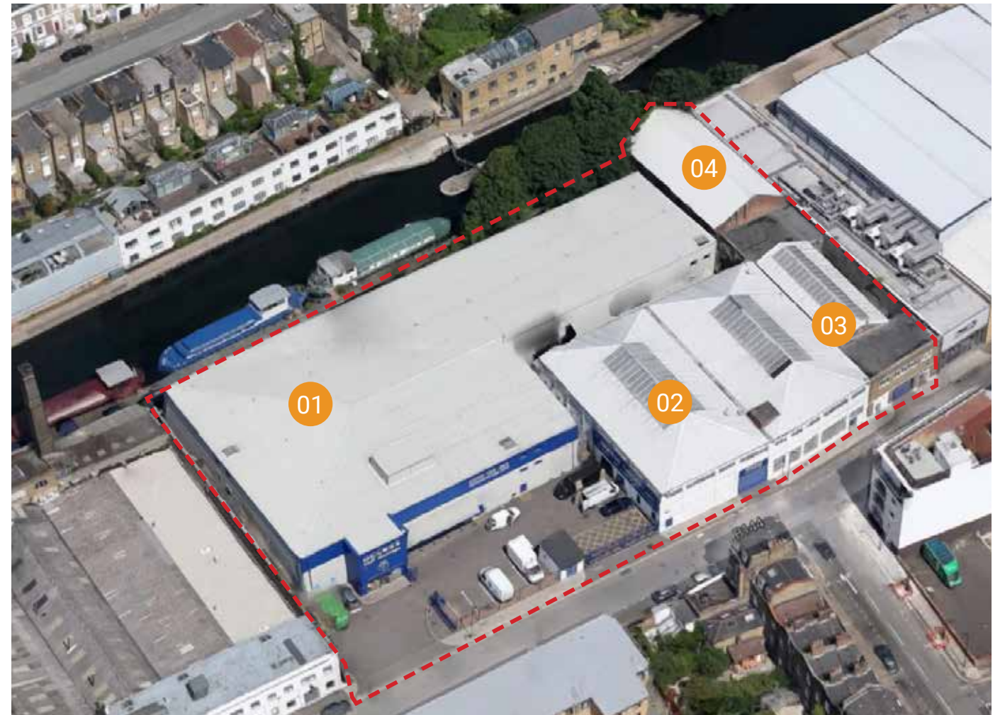
01 Light Metal Frame Building (1937) 02 Concrete Building (1937) 03 Brick Building (1965) 04 Victorian Brick Warehouse (c1860) with Polonceau Truss
