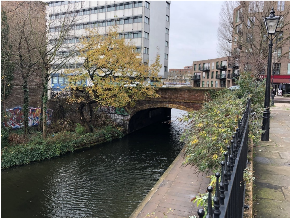
Figure 9 - looking west towards North Road Bridge over the Grand Union Canal
