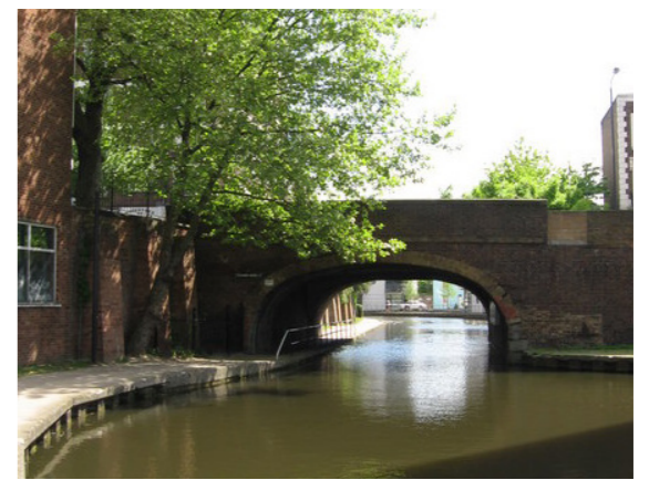
ref 2.12 North Road Bridge
