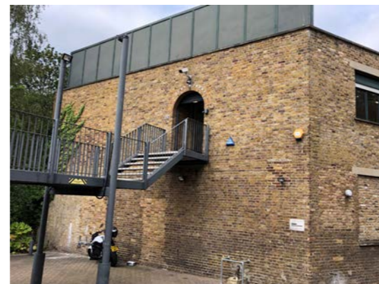
ref 2.25 View of existing site's adjoining building
