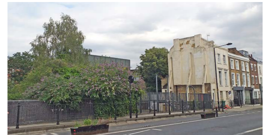
ref 2.35 Royal College Street Bridge
