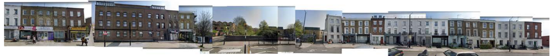
fig 2.29 Diverse east side brickwork styles, modern and traditional with a variety of buff brickwork and painted brick or painted render.
