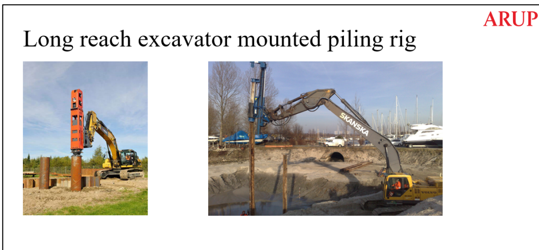
Figure 17 Typical Long Reach Piling Rig
