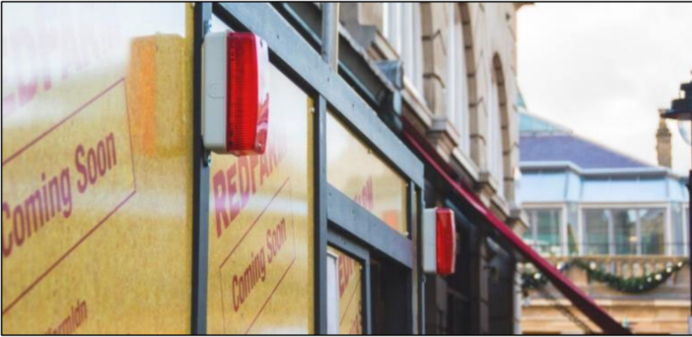
Figure 37 Typical hoarding lighting
