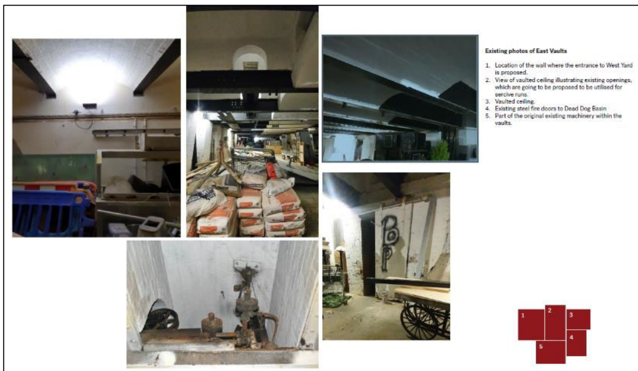
Figure 3 Existing photos of East Vaults
