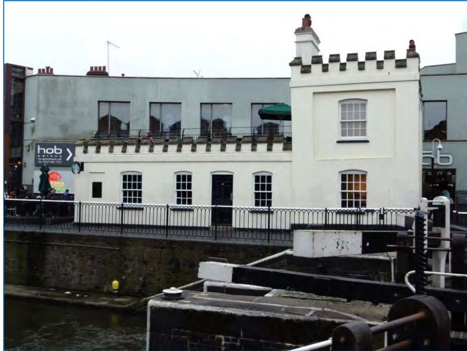
Figure 4.20: Regent's Canal information Centre
