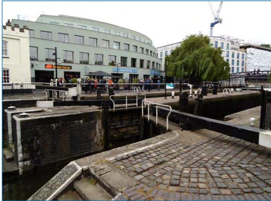
Figure 4.21: Hampstead Road Lock on the Grand Union Canal
