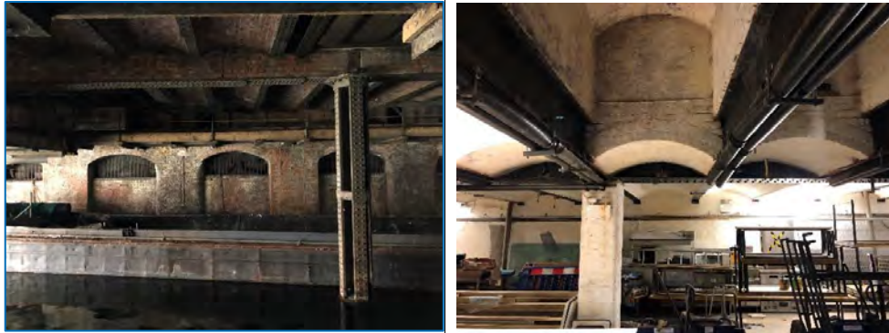
Figure 4.13: Dead Dog Basin (left) brick vaulted arches within basement (right)
