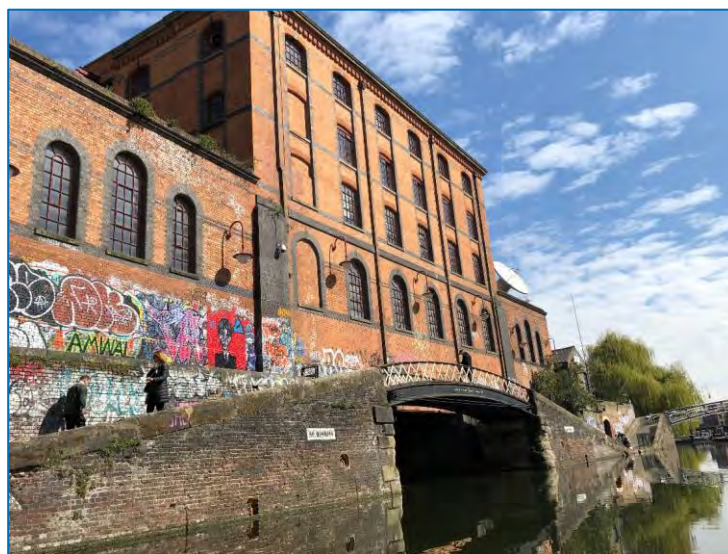
Figure 4.17: Towpath Bridge from Regent's Canal
