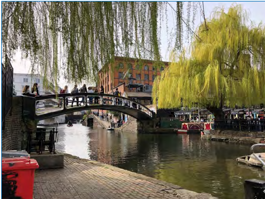
Figure 4.22: Roving Bridge from Regent's Canal
