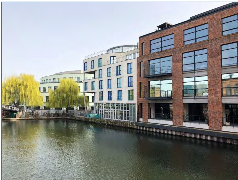
Figure 4.2: Modern apartment complexes to the south of the site across Regent's Canal
