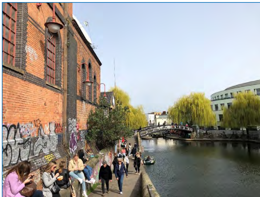
Figure 4.1: View of the Canal looking east from the interchange building
