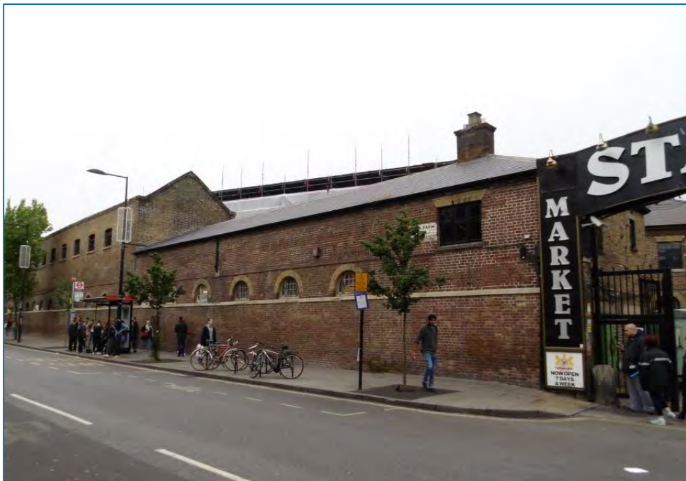
Figure 4.24: Stanley Sidings, Stables to east of Bonded Warehouse
