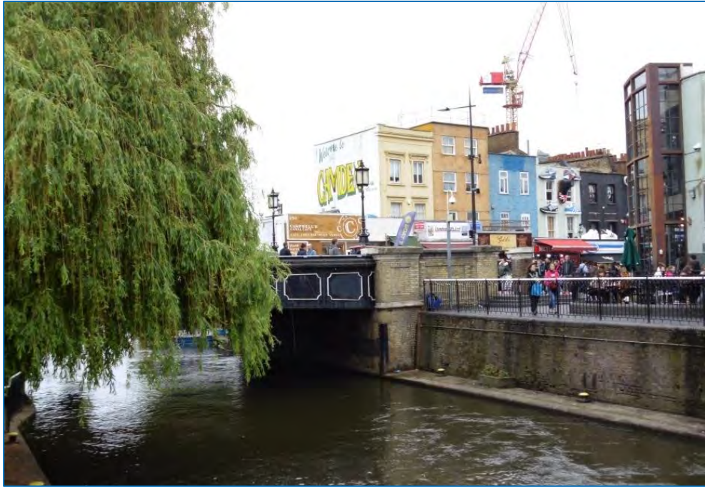
Figure 4.19: Hampstead Road Bridge Over Grand Union Canal
