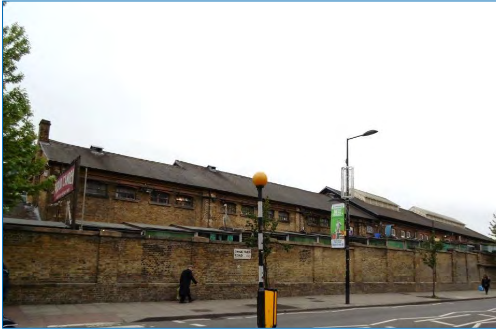
Figure 4.18: Horse Hospital with ramps and boundary wall at north of site
