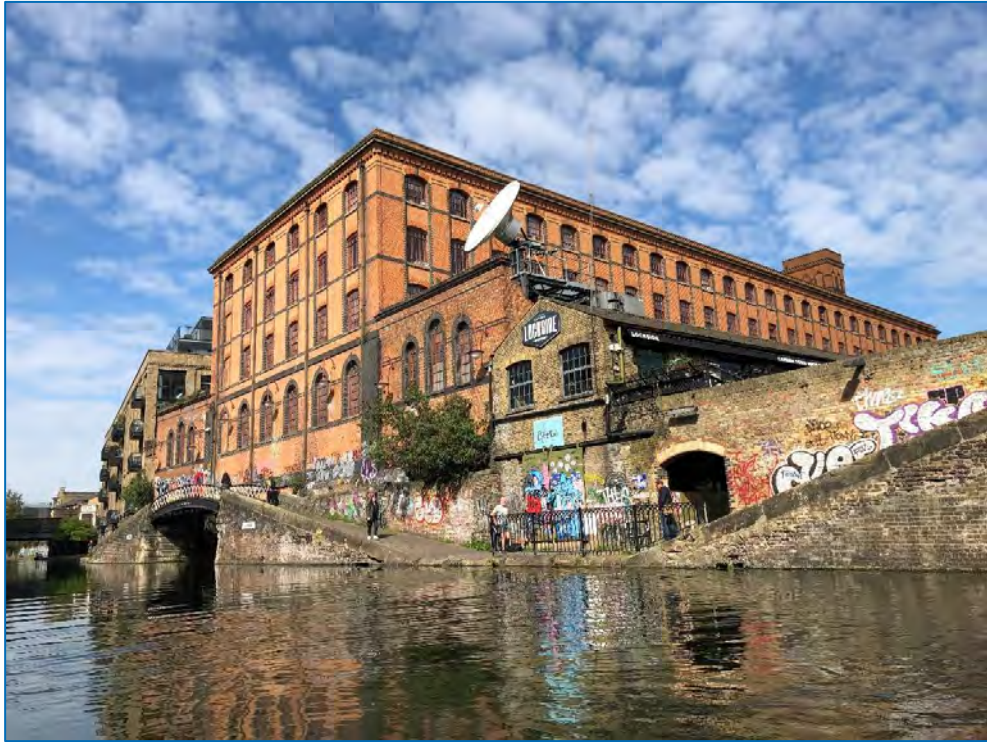
Figure 4.12: Interchange Building, as seen from Regent's Canal
