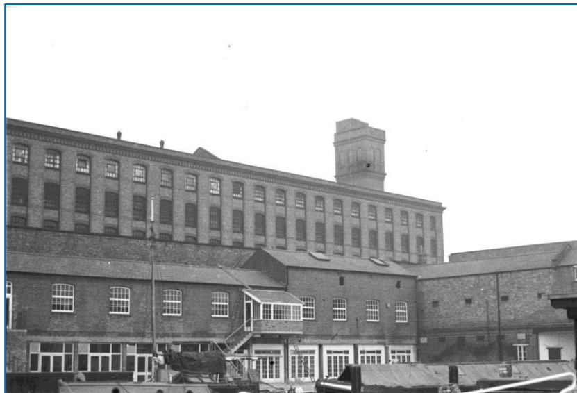
Figure 3.11: Photo dated 1973 of the Interchange and range of buildings in the west wharf
