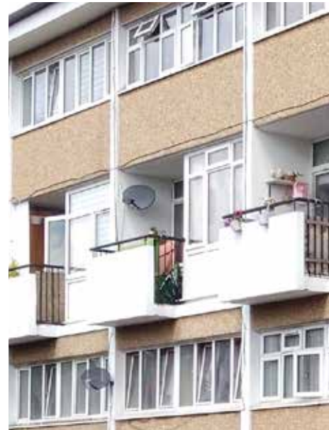
Semi-inset balconies, New Barnsbury
