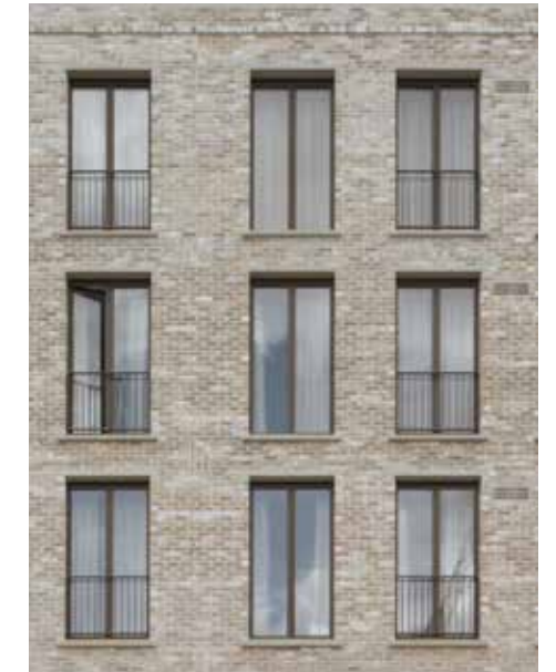
Equally proportioned and set out openings North West Cambridge, Witherford Watson Mann Architects
