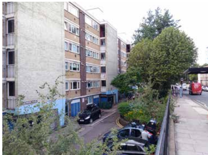
Blackmore House site levels fronting Copenhagen Street
