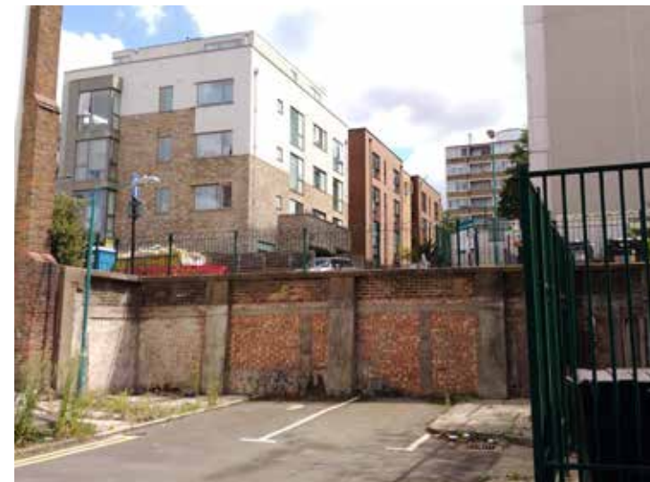
Blackmore House site levels fronting Copenhagen Street
