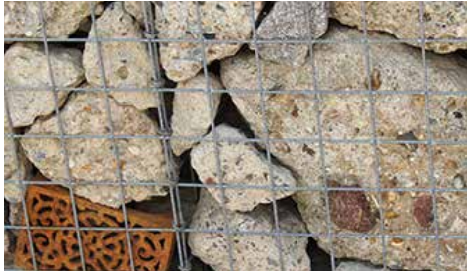
Rubble from demolition to be used for the Gabion Wall
