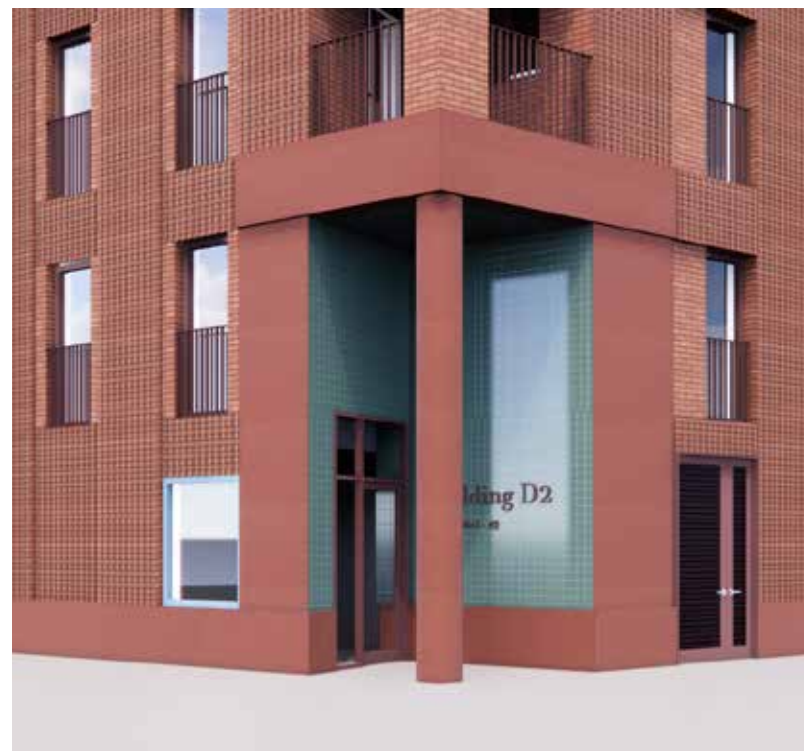
Double height communal entrance details marking the corner
