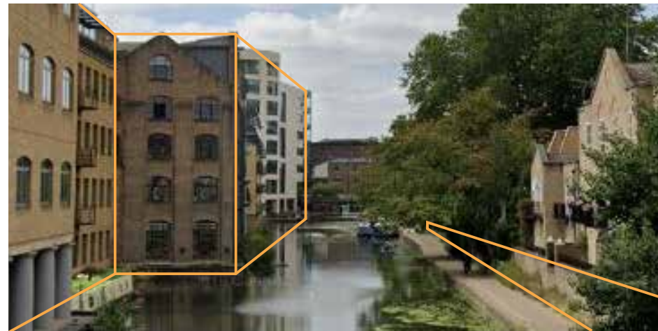
Thornhill Bridge looking west
