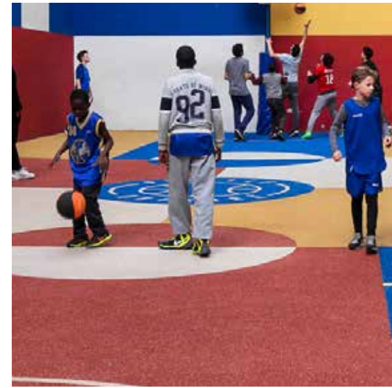
Sound absorbing surface to MUGA
