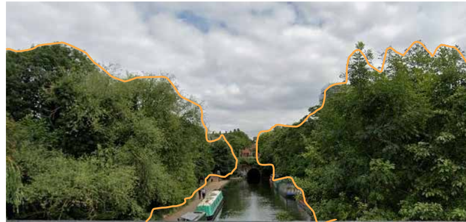
Thornhill Bridge looking east
