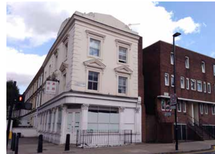
214 Caledonian Road, Copenhagen Street frontage
