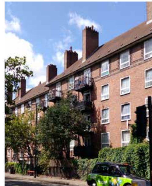
Old Barnsbury Mansion Blocks
