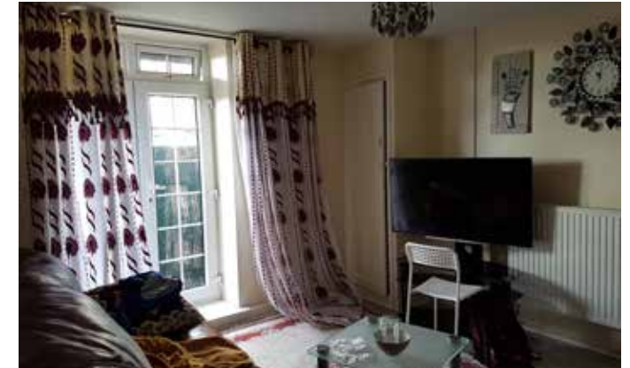
Problems with damp, noise, drafts and heat loss
