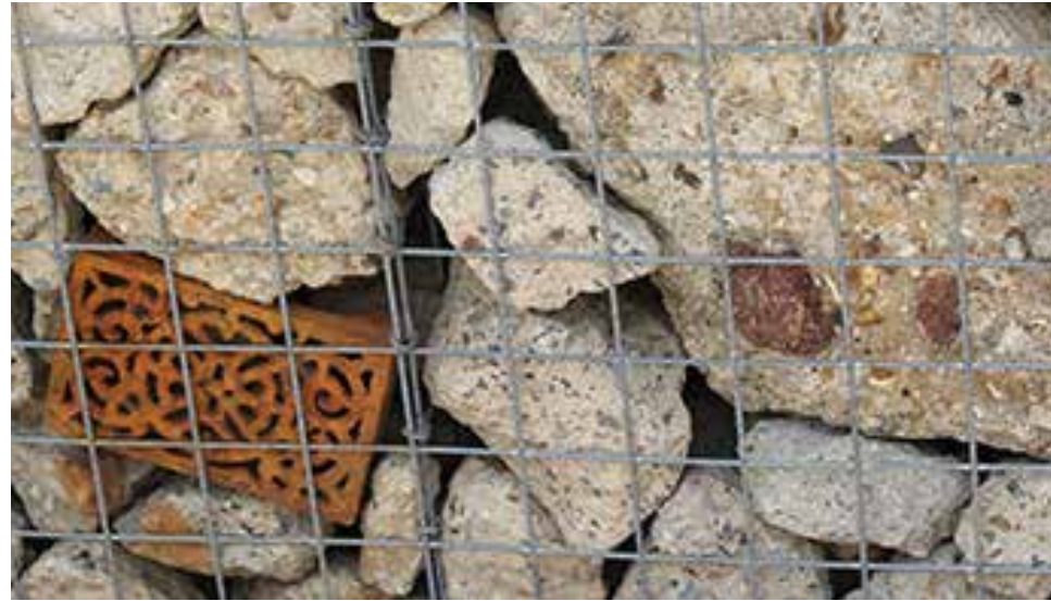
Reconstituted materials to create a Gabion Wall
