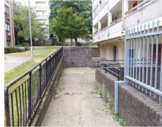
02. Levels at the rear of Messiter House
