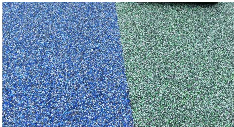
Wet pour safety surface to terraces and play equipment
