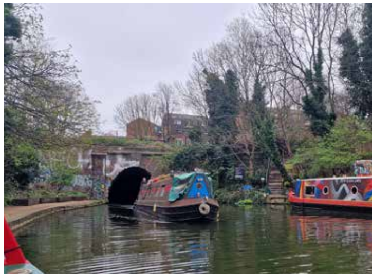
View from canal barge on approach to west portal
