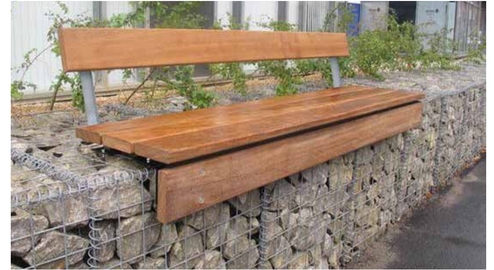
Gabion wall seating
