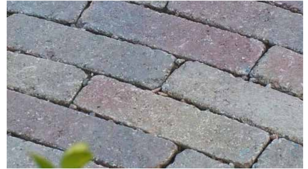
Entrance thresholds: Concrete brick paver Colour: Varies Mono-size: 200 x 50 (60mm thick) Pattern: Stretcher
