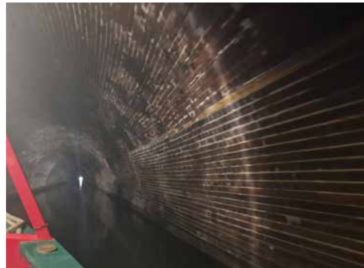
View from inside tunnel western portal side
