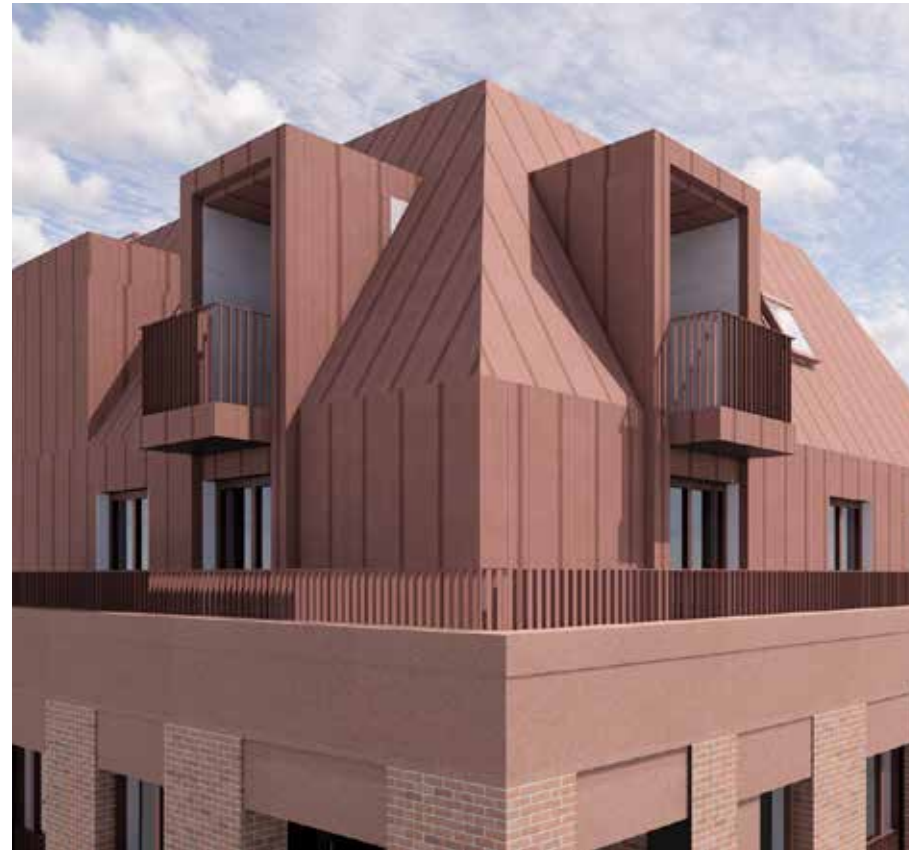
Mansion Block Metal Roof and Dormers
