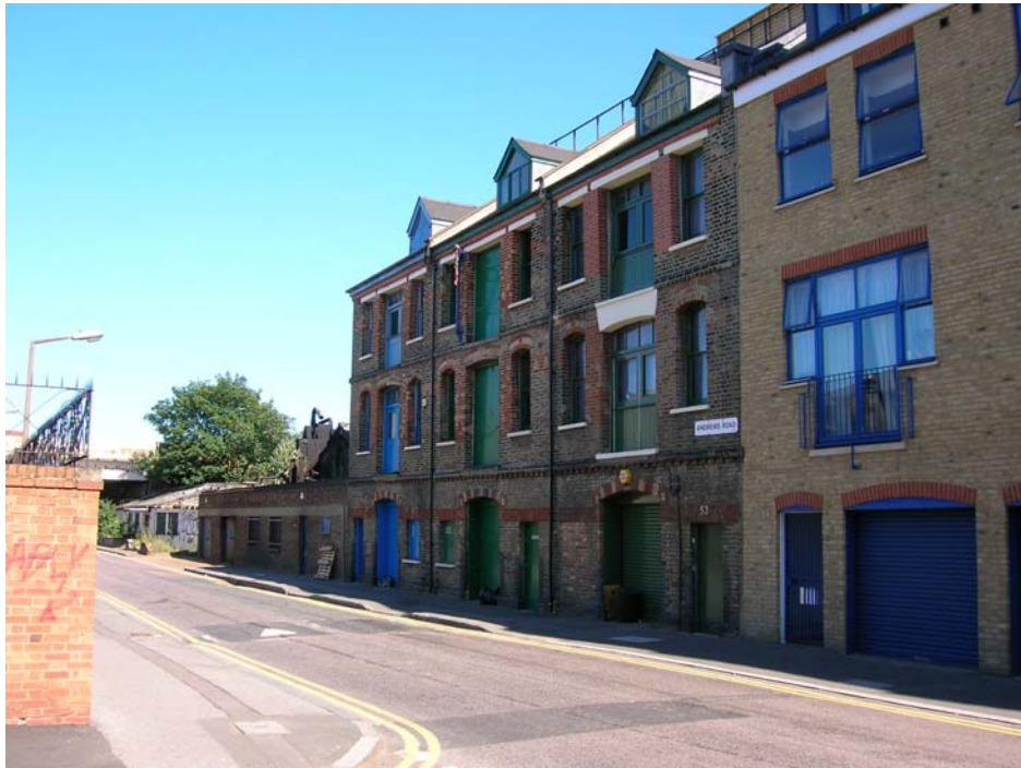
Fig. 16: South side of Andrews Road with Beehive Foundry to left and former factory/warehouses
