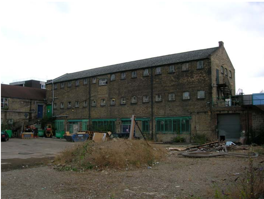
Figs 28 & 29: No.16 Hertford Road (former stable buildings)
