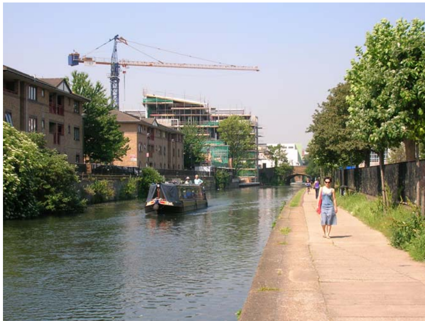
Fig. 1: General view of the Regent's Canal looking towards Queensbridge Road Bridge
