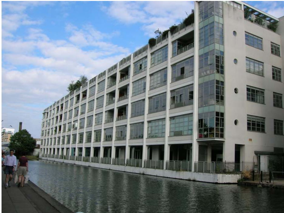
Fig. 4: Lofts at the former Royle Card Factory, at the junction of the Regent's Canal and Wenlock Basin
