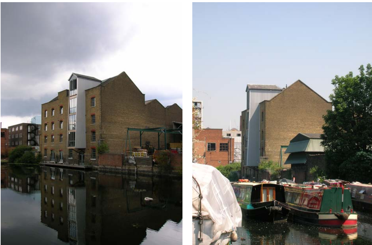
Fig. 26: Two views of the refurbished Quebec Wharf (Spice Warehouse)
