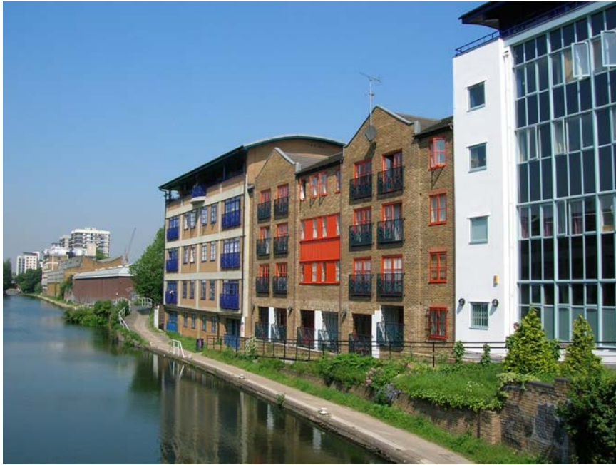
Fig: 24: New developments between Kingsland Bridge and the entrance to the Kingsland Basin
