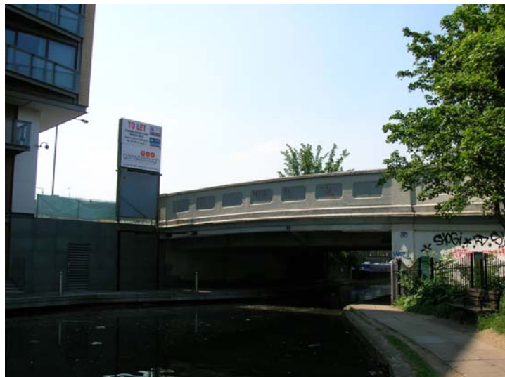
Fig. 41: New North Road Bridge
