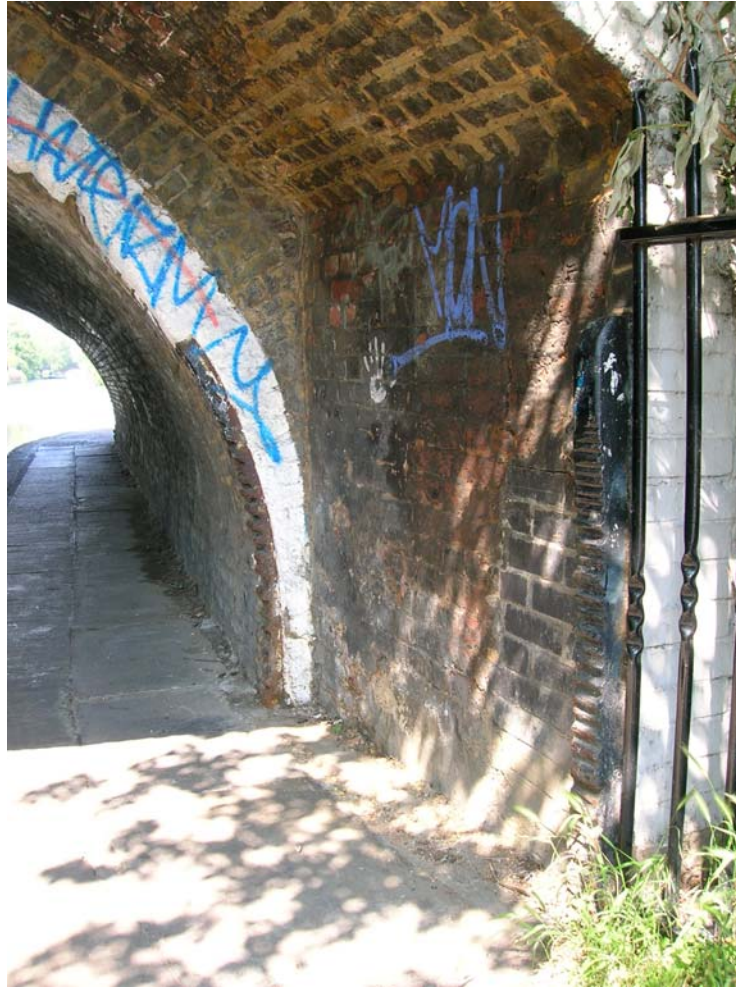
Figure 49: Deep grooves in the cast iron rubbing strips made by ropes of horses
