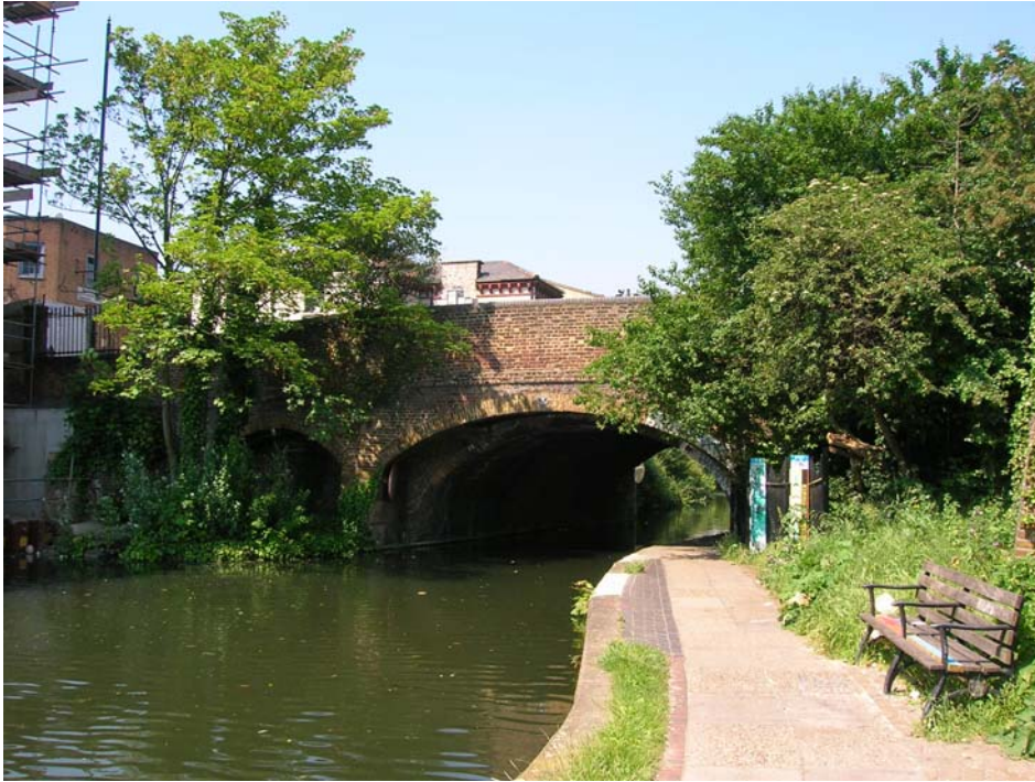
Fig. 23: Kingsland Road Bridge, showing improvements to bridge corners
