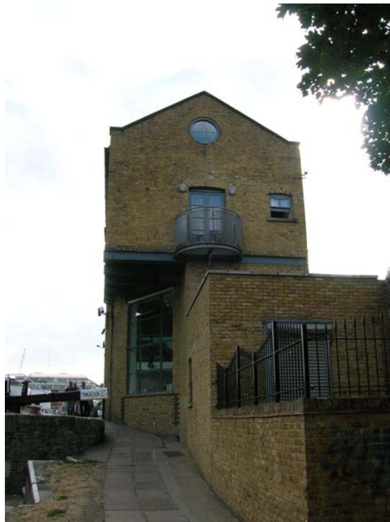
Fig. 48: Refurbished Lock Keepers Cottage and Pumping Works at Sturts Lock
