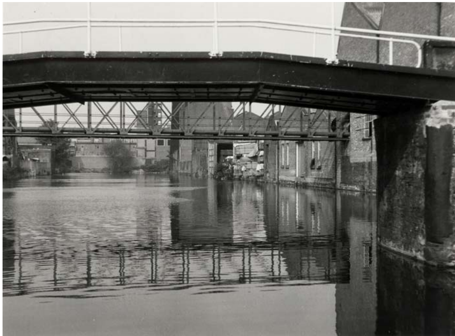
Fig. 25: Entrance to the Kingsland Basin in 1950s (iron pedestrian bridge now removed)
