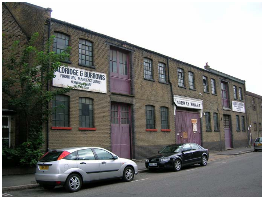
Fig. 27: Norway Wharf (Nos. 18-20 Hertford Road)
