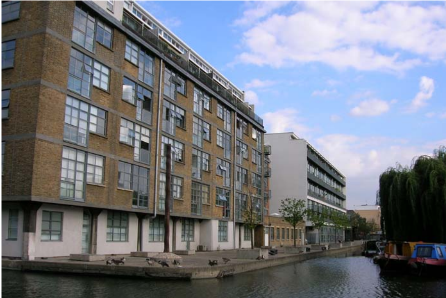
Fig. 46: Looking south along Wenlock Basin
