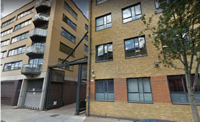
Ice Wharf South east facing windows
