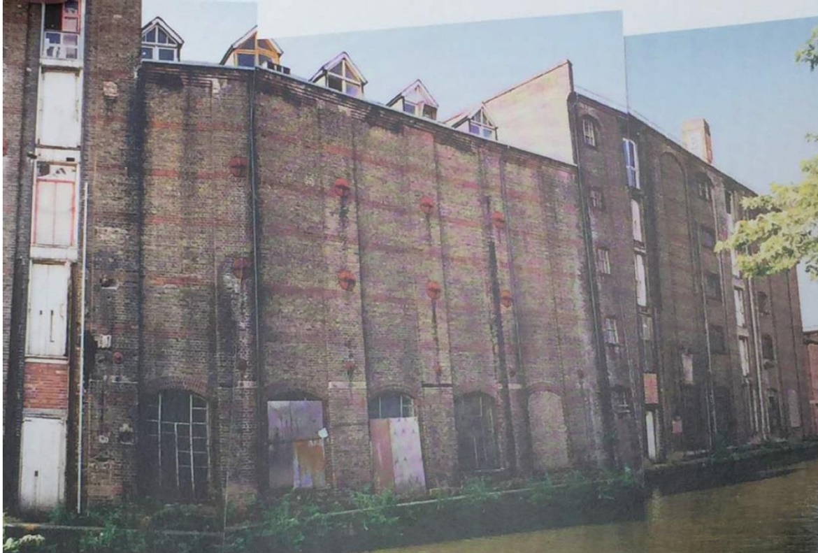
No. 10 Regents Wharf prior to renovation
