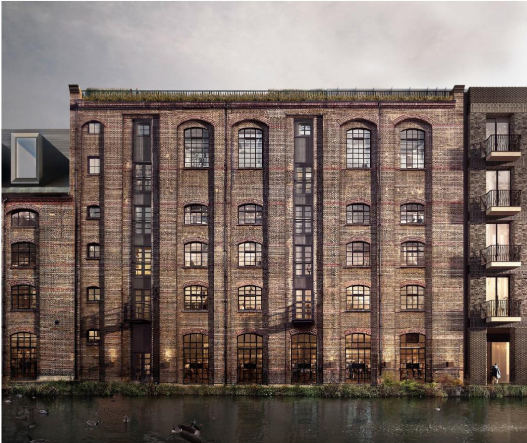
Building B (No. 12 Regent's Wharf) – canal-side elevation
