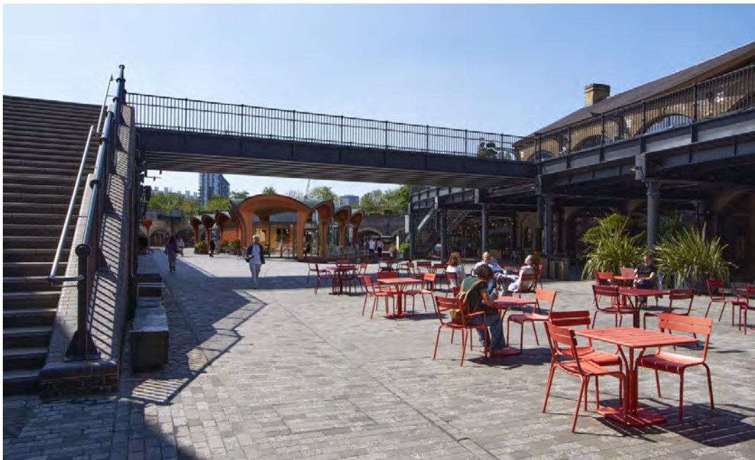
Fig 46: CGI of the Pavilion as viewed from the North at Yard level with Wharf Road Viaduct (now Bagley Walk) and Camley Street Natural Gardens beyond.
