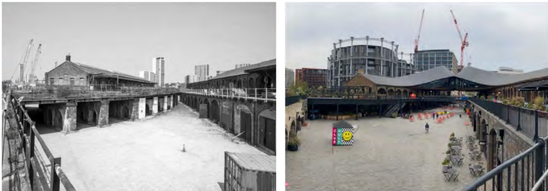
Figs 18 & 19: Coal Drops Yard in 1989 (left) and today (right), showing the removal of the Plimsoll Viaduct to reveal the earlier Western Viaduct and to enable the creation of a strong north-south circulation between the remaining viaducts at yard level.
