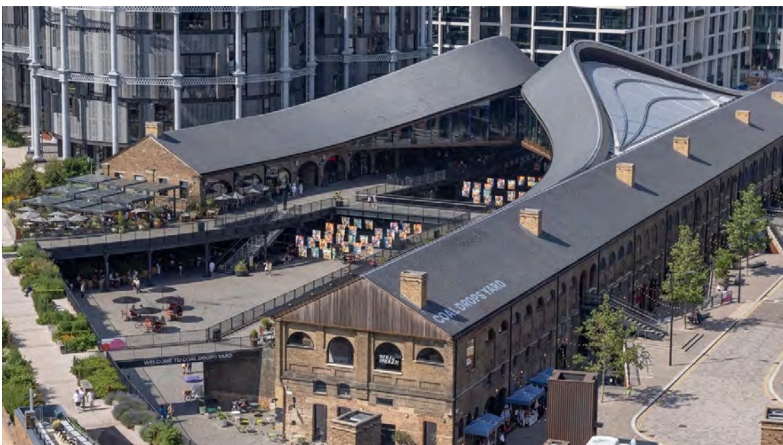
Fig 20: Aerial view of Coal Drops Yard today looking north-west, showing the enlarged southern yard and the sweeping new 'ribbons' at roof level
