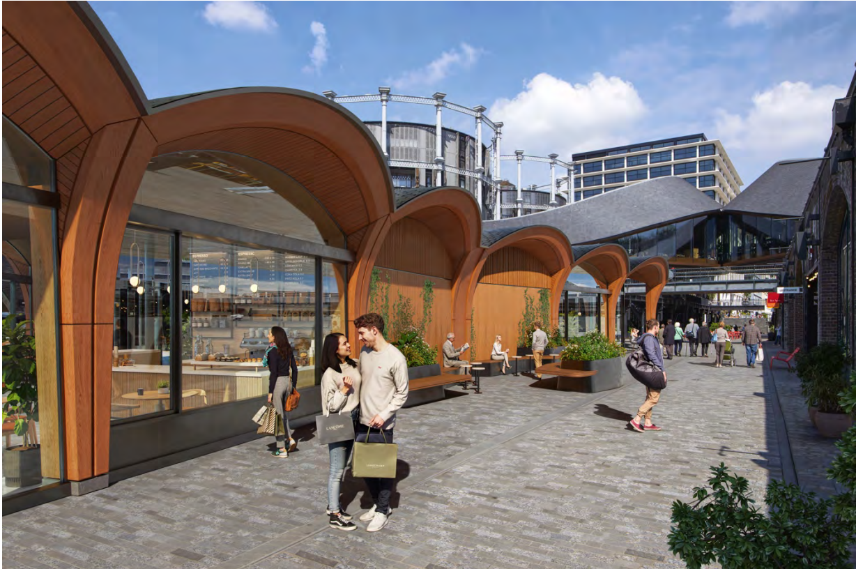
Fig 49: CGI view of the eastern elevation of the pavilion looking north to the Heatherwick 'ribbons' and with the Easter Coal Drop Viaduct directly opposite.
