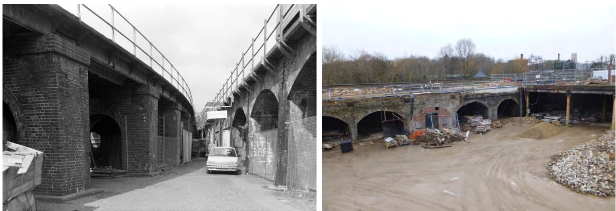
Fig 17(L): The Plimsoll Viaduct (left) in 1989 looking north at the junction with the East Coal Drop Viaduct (right)
