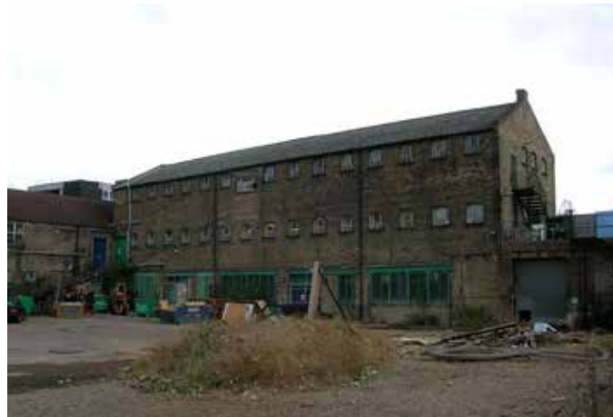
Hertford Road (former stable buildings)
