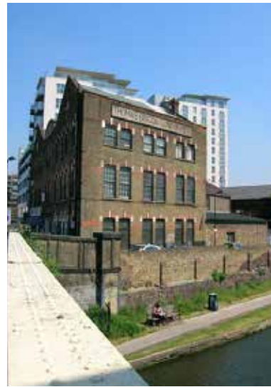
Thomas Briggs Factory and Rosemary Works by Rosemary Branch Bridge
