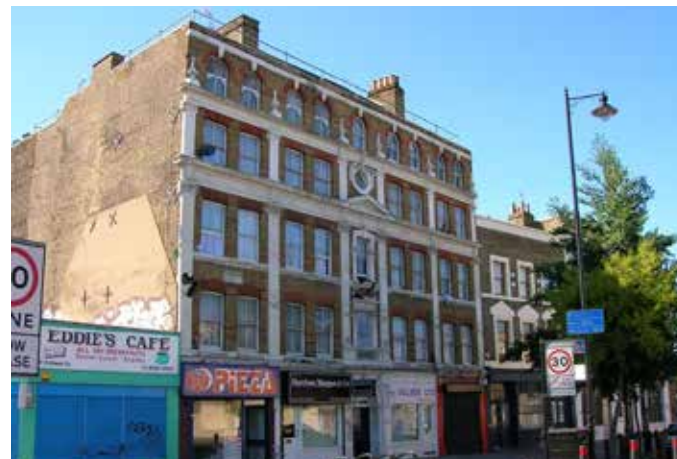
Mare Street (Locally Listed Building)
