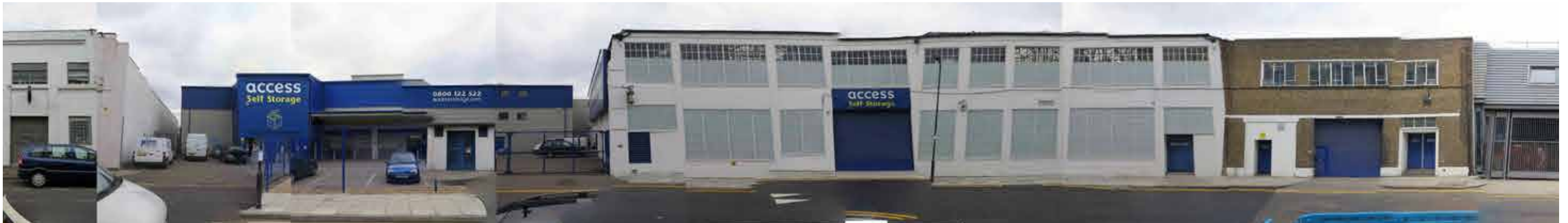
Eagle Wharf Road Elevation
