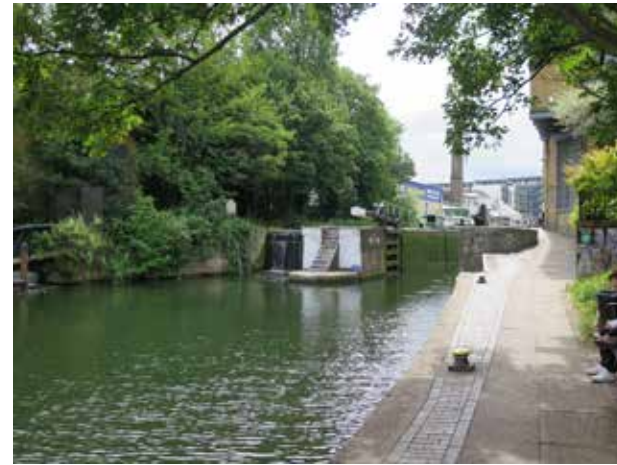
1. Looking West along Regent's Canal, Sturt's Lock
