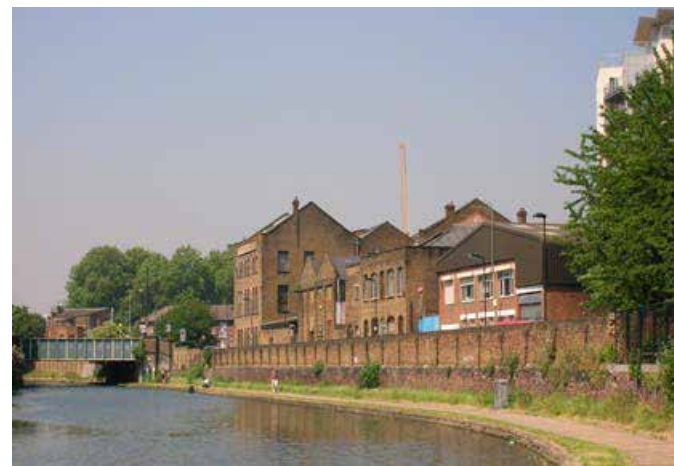
View westwards from Whitmore Bridge
