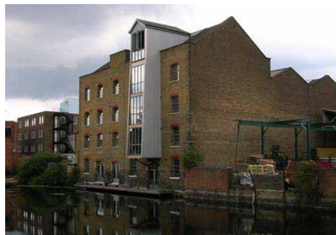
Refurbished Quebec Wharf (Spice Warehouse)
