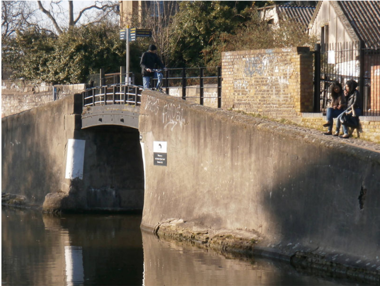
The Stop Lock bridge and towpath
