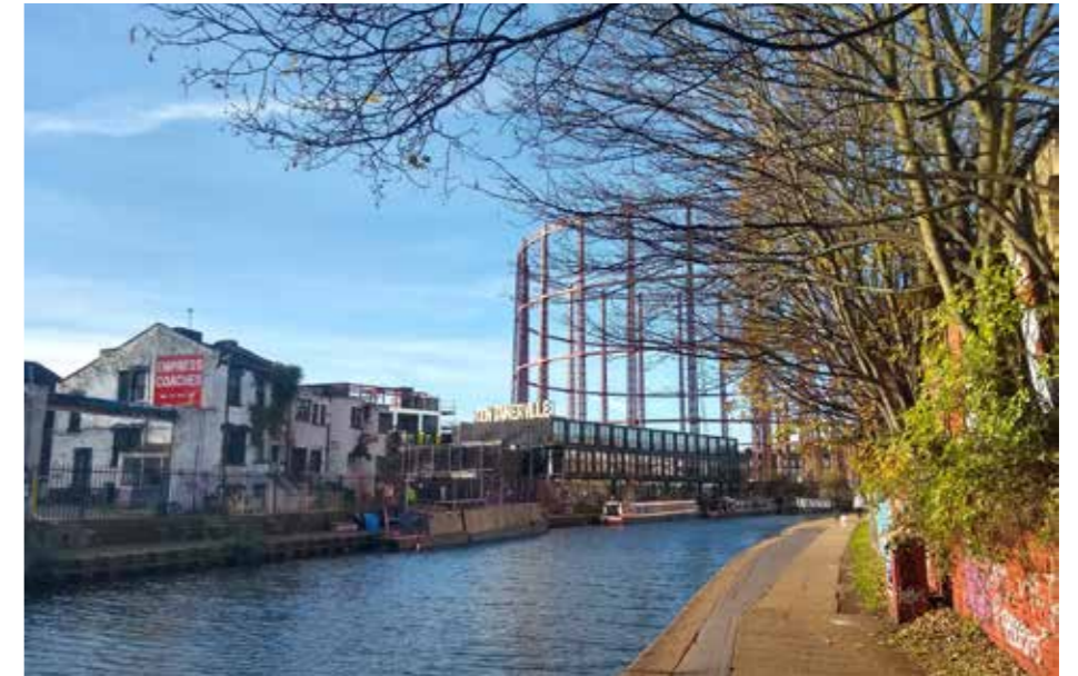
Figure 4.4 View from close to Mare Street bridge
