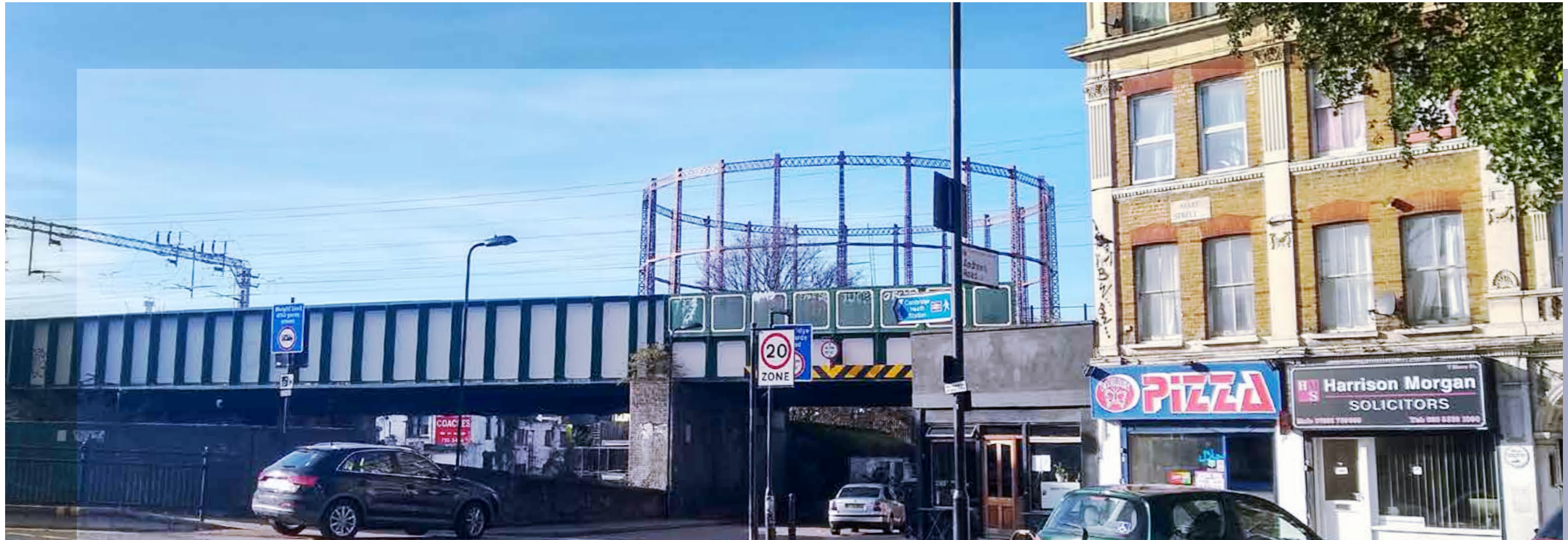
APPENDIX 2: Marian Place Gas Holder Station Bethnal Green English Heritage Coil Advice Report (2015)
