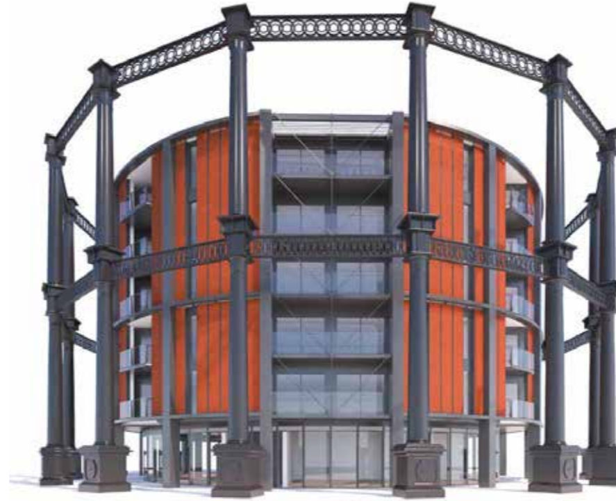
Figure 6.3 Illustration of the elevational treatment of Building E showing how the rhythm of the bays interrelate to that of the gasholder frame.
