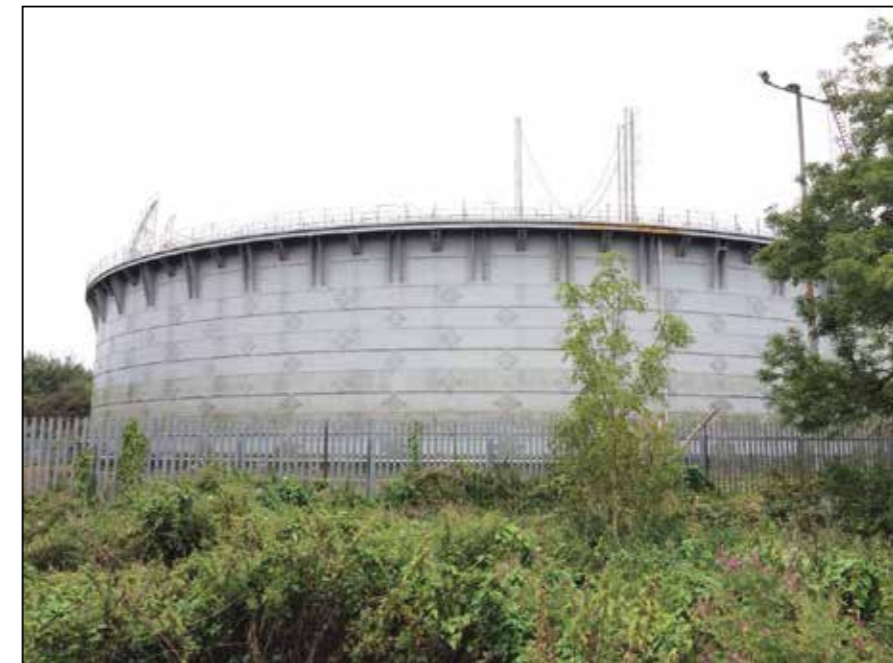
Figure 1.2: Photograph of a spiral guided gasholder with an above ground built in 1930.
