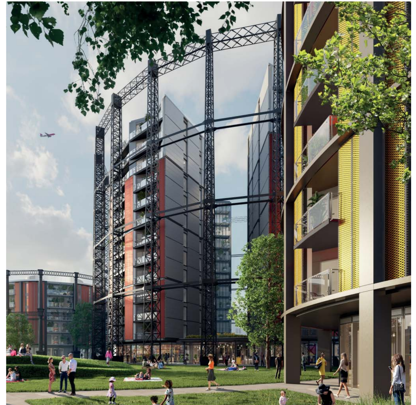
Figure 5.2 Space between and within gasholders
