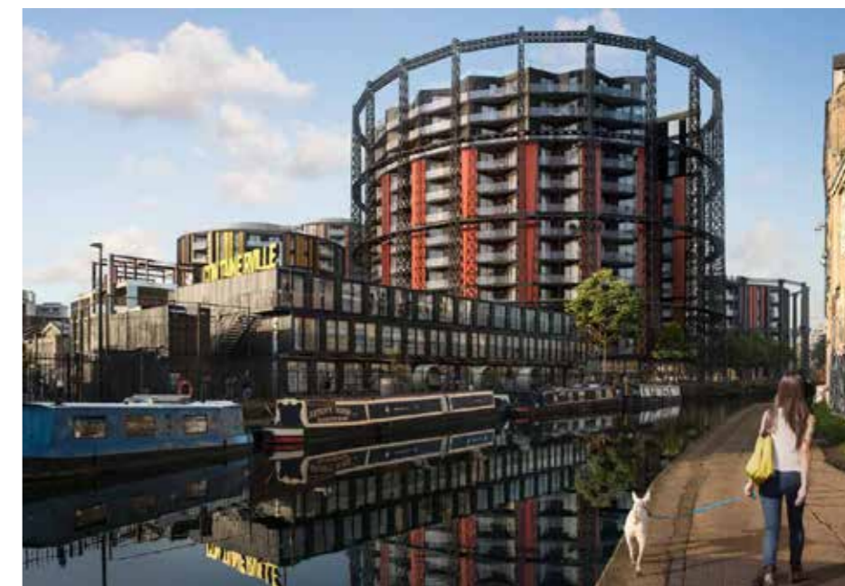
Figure 6.2 CGI showing the retention of the existing gasholder frames with new buildings inside, taking from the Regent's Canal.
