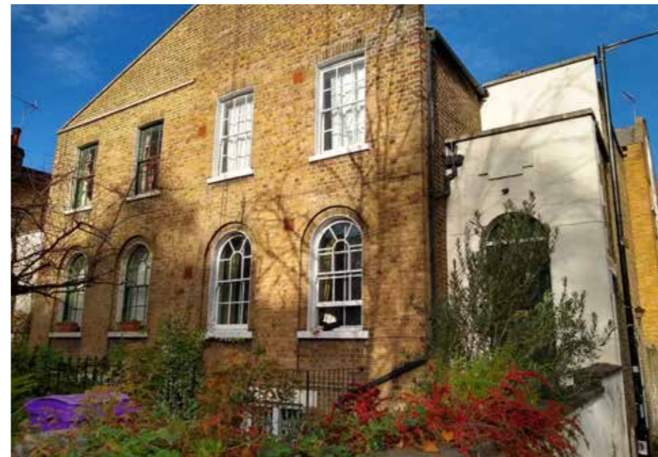
Figure 4.10 369-371 Hackney Road, which form part of the terrace of pairs at 363-373
