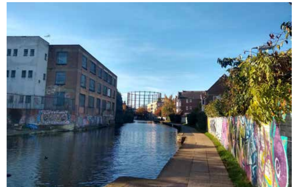
Figure 4.5 View from beyond Mare Street Bridge towards the gasholders
