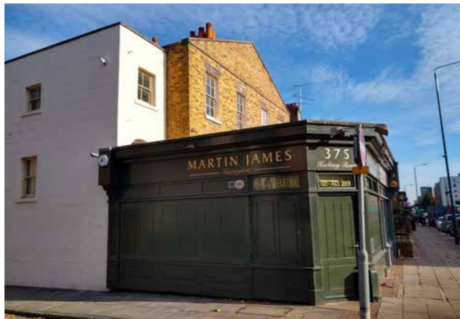
Figure 4.9 Corner of 375 Hackney Road
