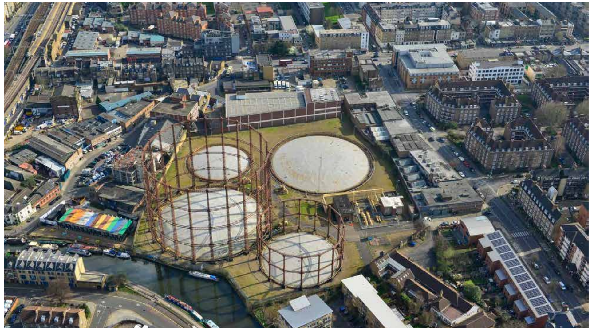
Figure 0.1 Aerial photograph showing the location of the former gasholder site at Marian Place facing south.
