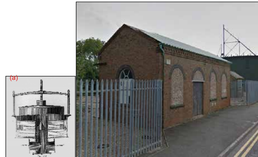
Figure 1.6: (a) Station Governor from King's Treatise on Gas (1879); (b) An example of a governor house.
