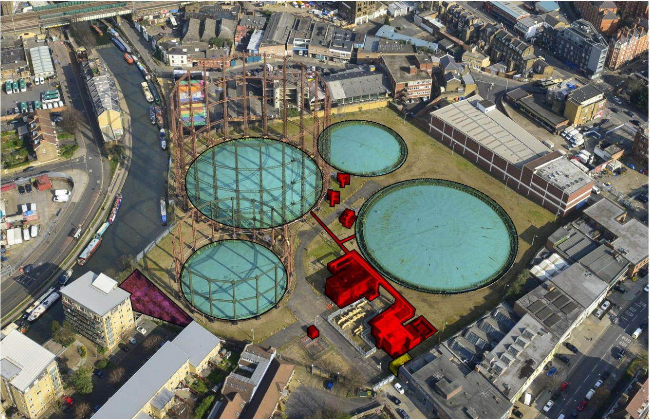
Figure 3 - Coloured items to be removed - Redundant Gas Infrastructure (Red), Gasholder Metal Tanks (Turquoise), Substation Housing (Yellow), Concrete Hardstanding (Purple)
