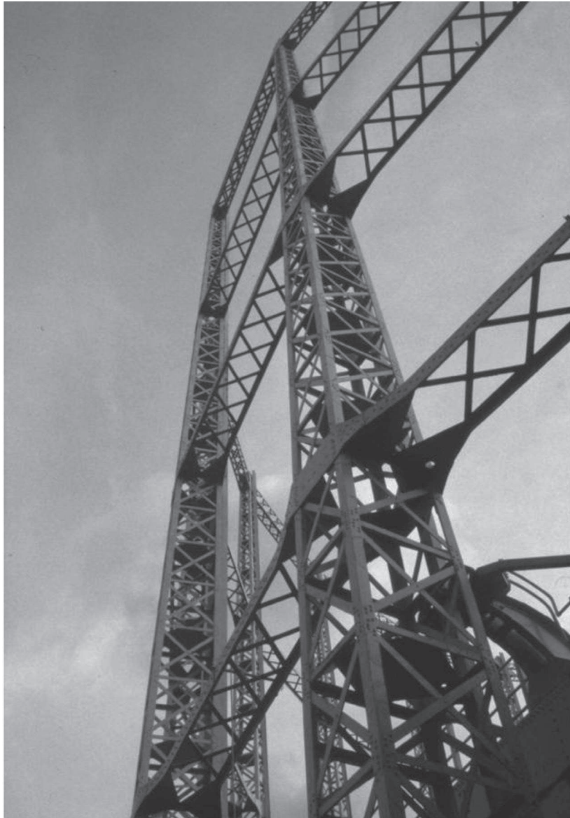
Bethnal Green Gasholder No.5 constructed 1889
