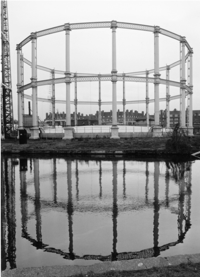
Bethnal Green Gasholder No.2, constructed 1866
