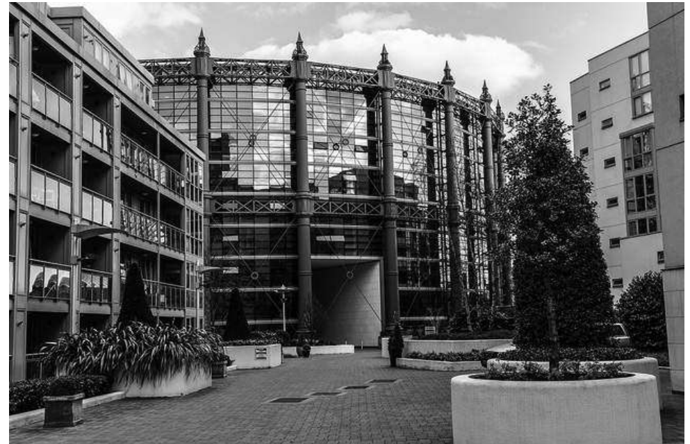
Figure 3: The Alliance Gasholder, Dublin Docks
