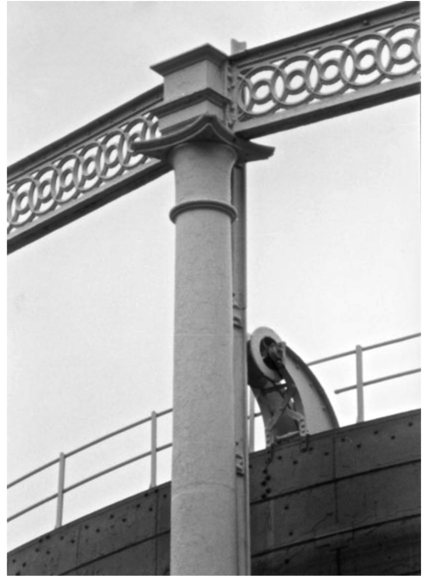
Detail of Bethnal Green Gasholder No.2
