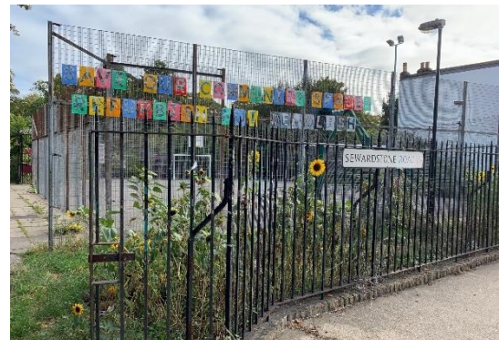
SEWARDSTONE ROAD FRONTAGE
