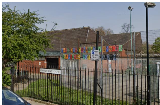
EXISTING BUILDING ON THE SITE
