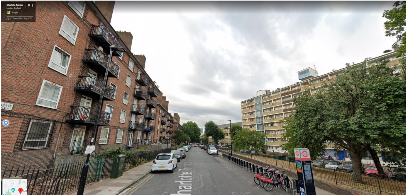
Photo 20: Charlotte Terrace looking south with New Barnsbury to the right and Old Barnsbury to the left
