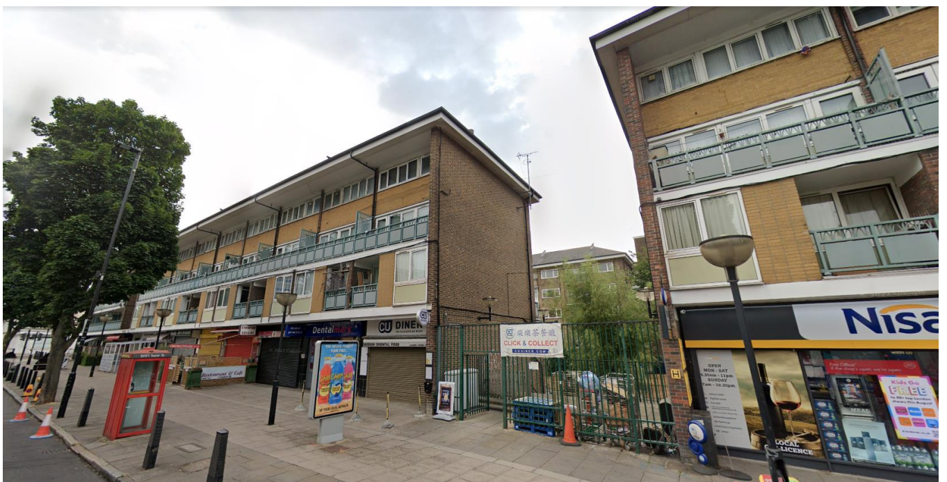
Photo 5: Mid point of Caledonian Road frontage
