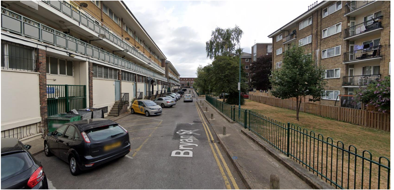
Photo 8: Rear of Caledonian Road, looking north to Copenhagen Street along Bryan Street.
