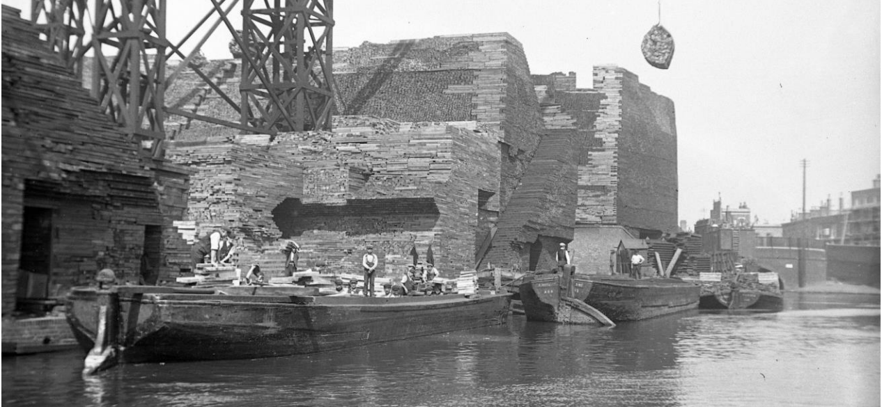
Photo: Timberyard looking West from Whitmore towards the Rosemary Branch, 1907, London Canal Museum
